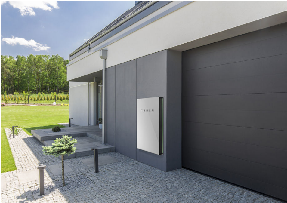
Figure 3. Example of a Powerwall Installed on a House
