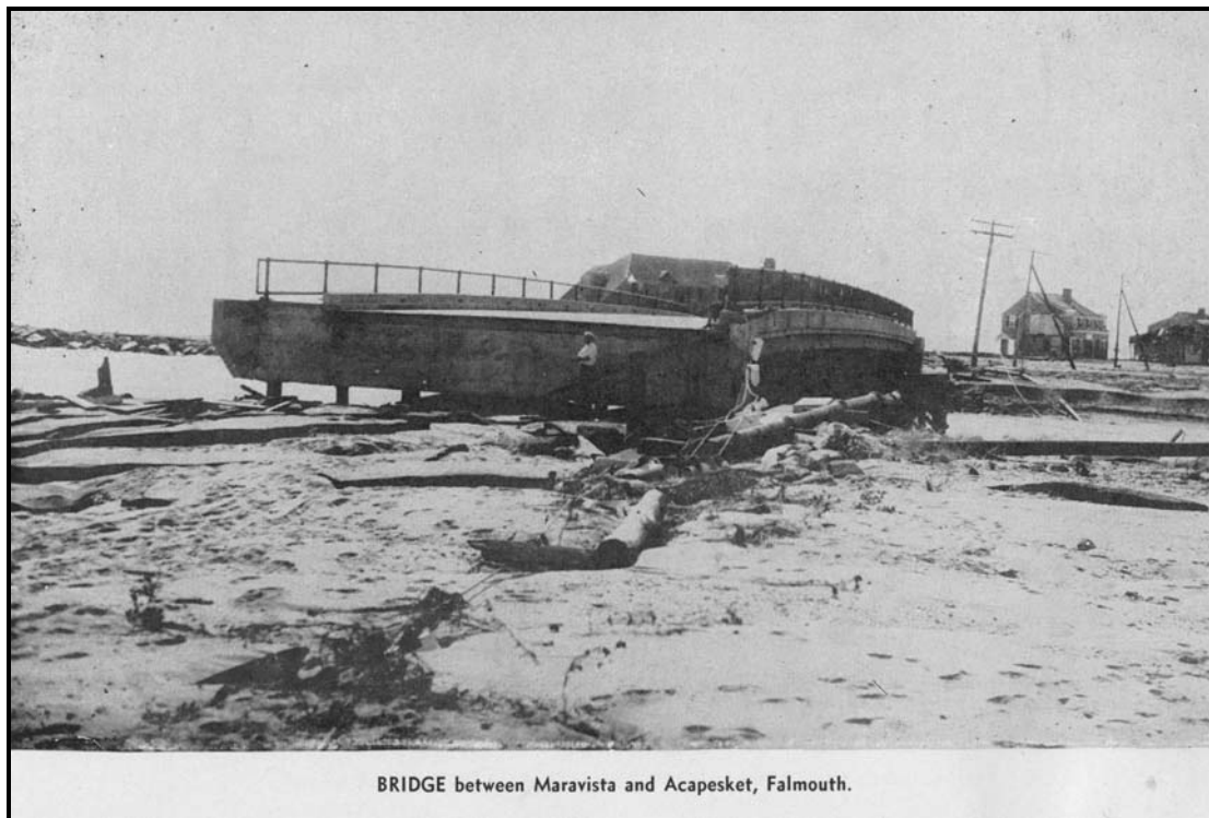
Figure V-8. Photograph of the old Great Pond bridge immediately after the 1944 Hurricane. The photograph shows that storm overwash eroded the roadway and approach ramps to the bridge. Note the Great Pond western jetty at the left side of the photograph.
