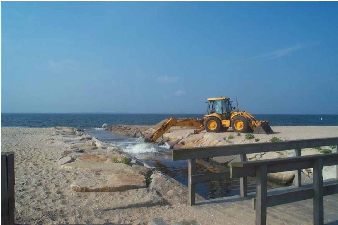
Figure V-4. Typical dredging required to maintain the Little Pond entrance channel.
