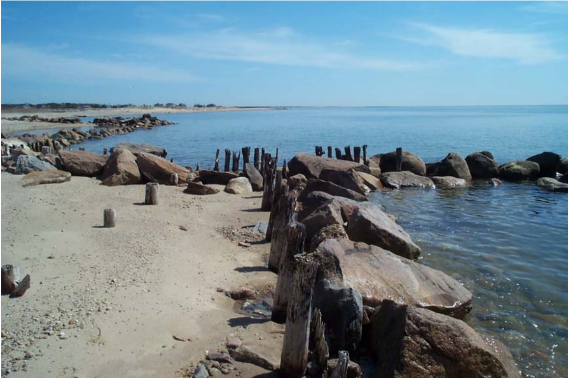
Figure V-7. Photograph of the shoreline west of Menauhant Beach taken in 2004 showing remnants of a timber bulkhead and groin, as well as more recent stone structures.
