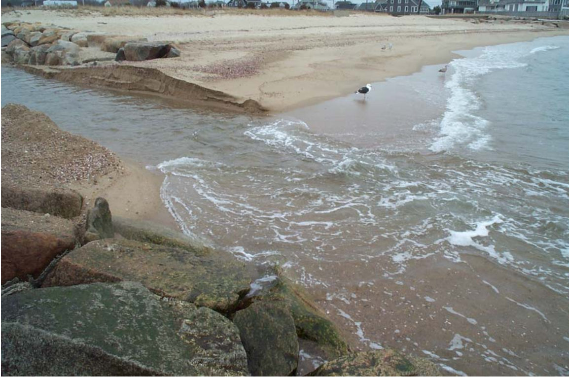
Figure V-3. Shoaling of the Little Pond entrance channel in 2004, where littoral drift caused beach sediment from the east side of the inlet to partially block the channel.
