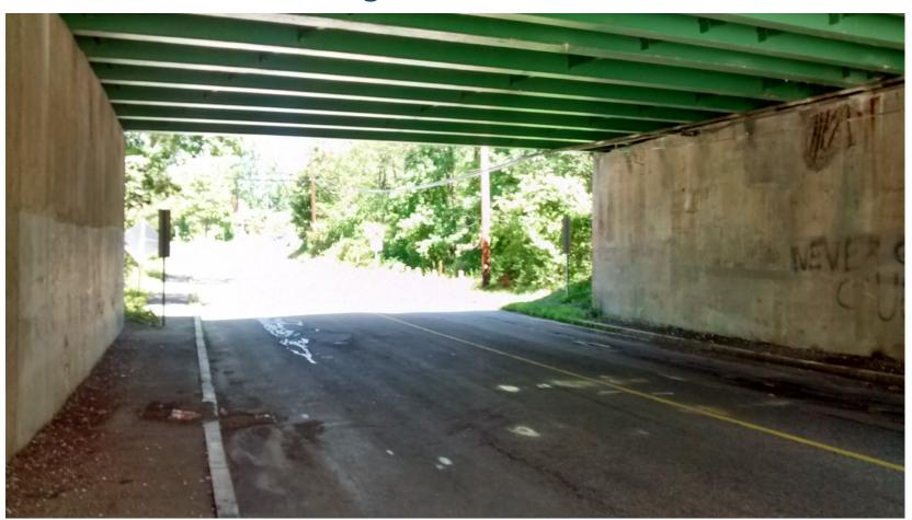
Route 2 Overpass – Looking northeast on Foster Street poor lighting / sight distance, lack of pedestrian & bike facilities
