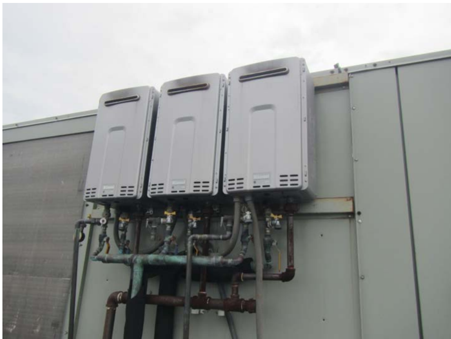
Direct gas-fired heating units on roof top AHU
