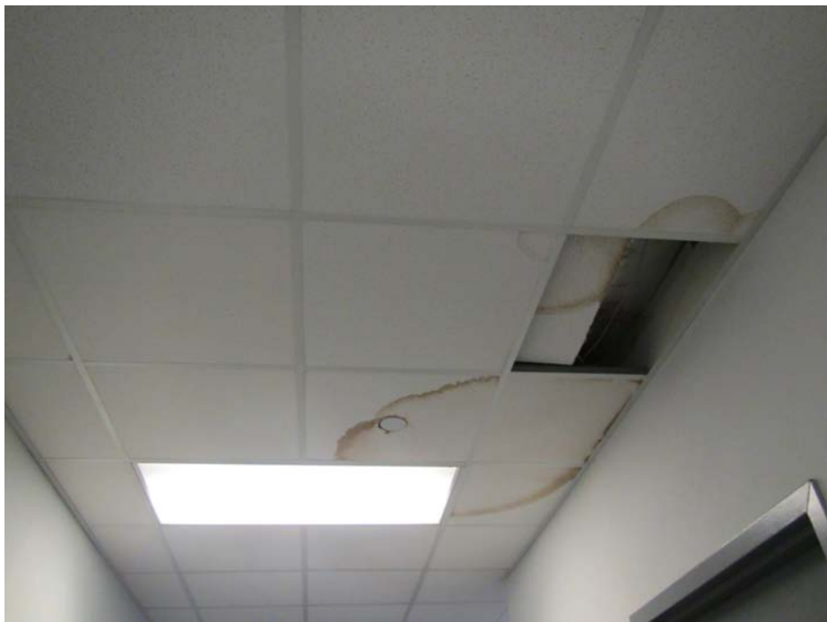
Water-damaged and missing ceiling tiles
