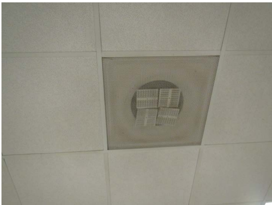
Ceiling-mounted supply vent
