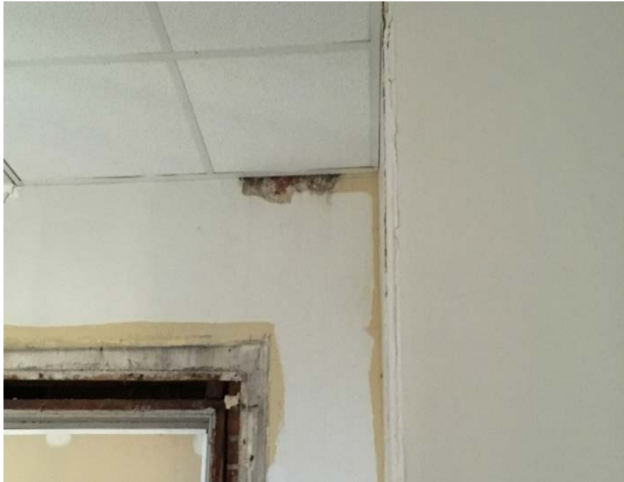
Mold staining on wall
