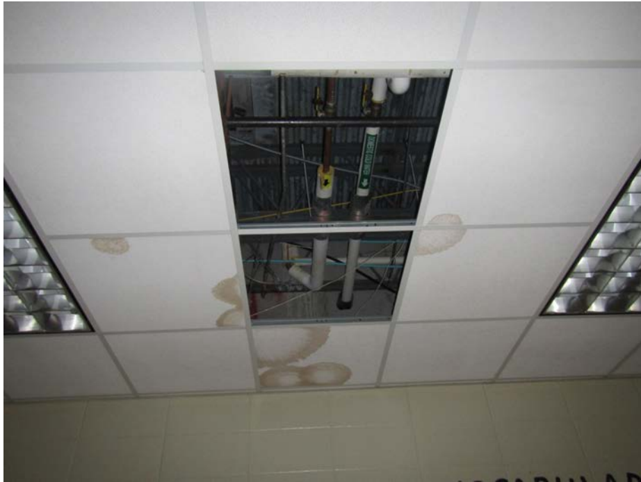
Water-damaged and missing ceiling tiles
