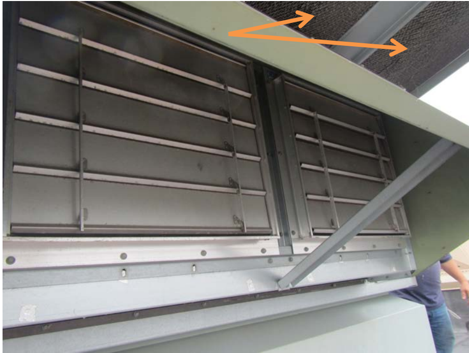
Fresh air intake vent (arrows) and closed exhaust louvres (below)
