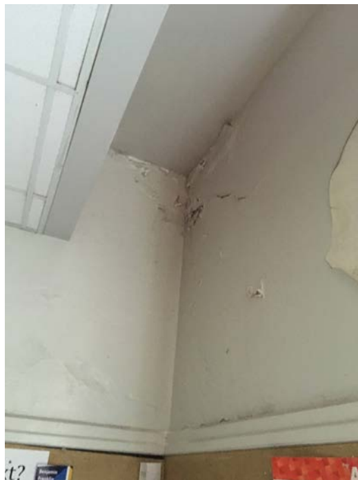
Water-damaged ceiling plaster
