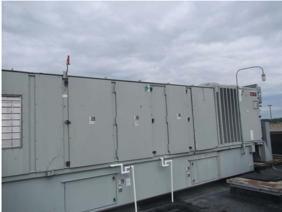
Large “packaged” AHU on the roof
