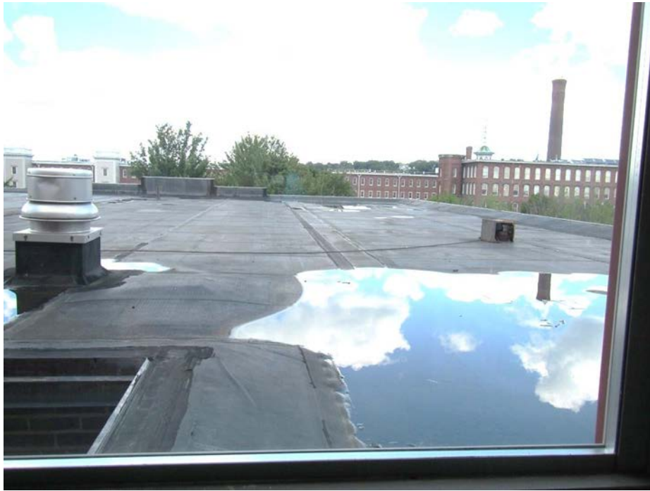
Water pooling on roof
