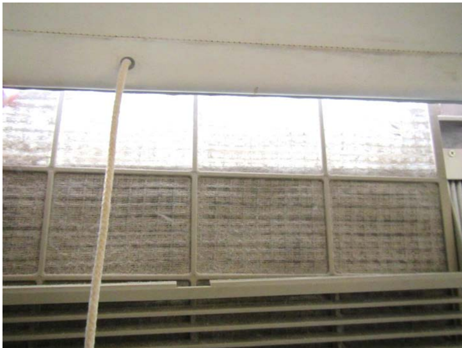
Very dusty window air conditioner filter
