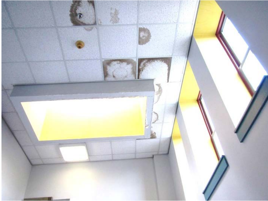
Water-damaged ceiling tiles next to skylight
