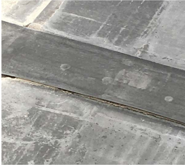
Detached roof membrane
