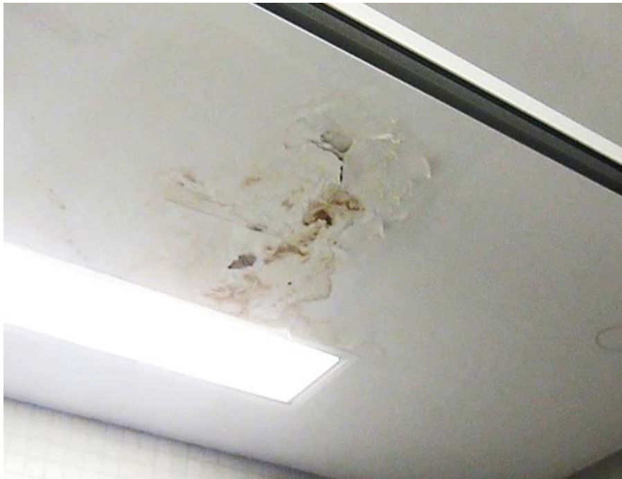
Water-damaged ceiling plaster
