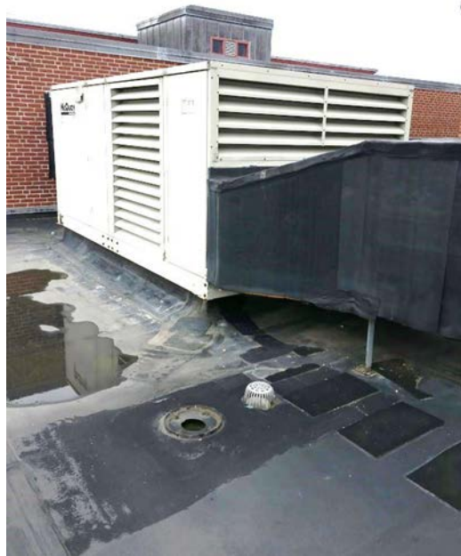
Rooftop air handling unit (AHU)
