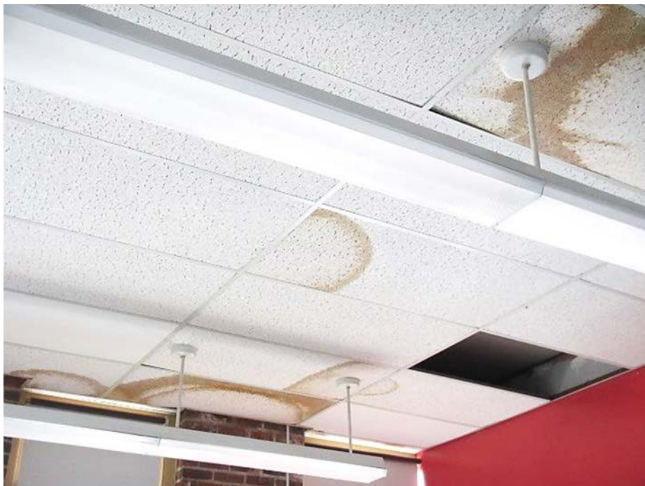
Water-damaged and missing ceiling tiles
