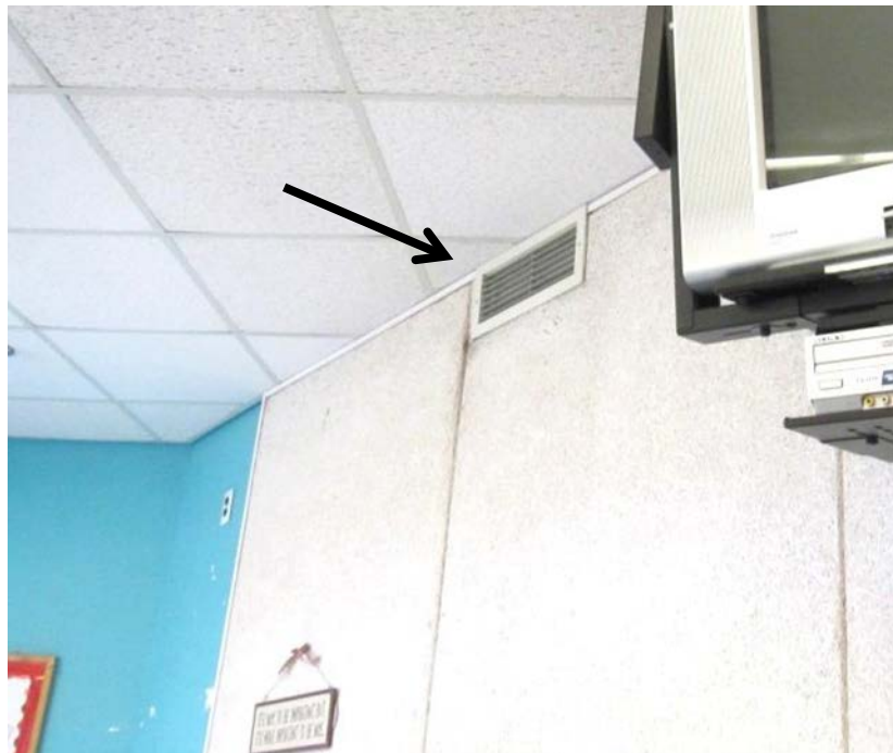
Wall-mounted supply diffuser (arrow)
