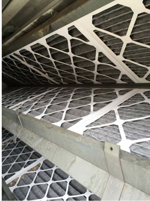
Bank of pleated filters in AHU
