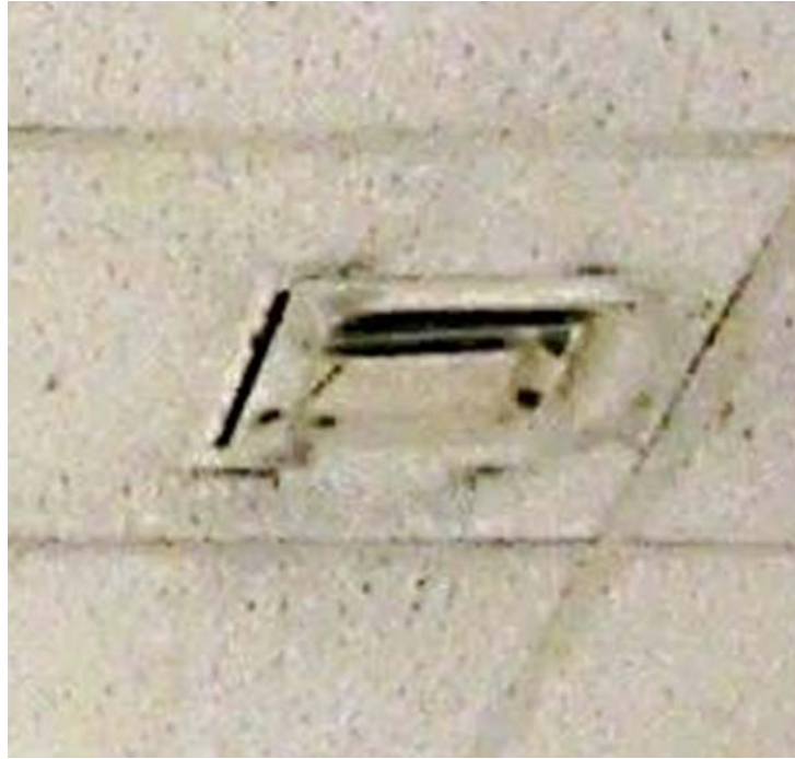
Ceiling-mounted supply diffuser, note accumulated dust/debris on louvers/ceiling tiles
