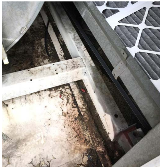
Dust/debris accumulation inside AHU
