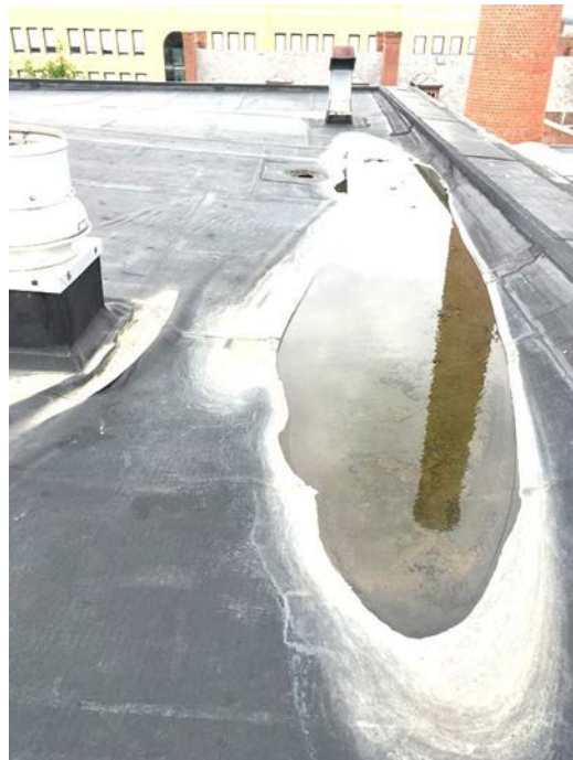
Water pooling on roof
