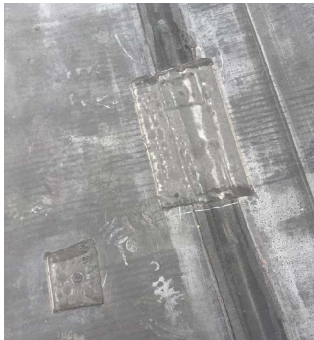
Detached roof patches
