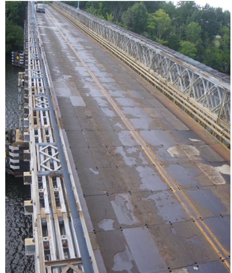
Existing Rourke Bridge
