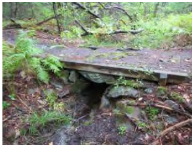
Stone Slab Bridge (DCR)
