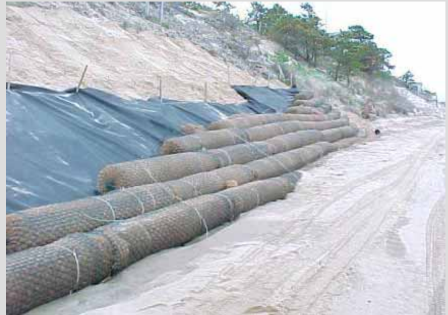
Fiber Roll Installation
