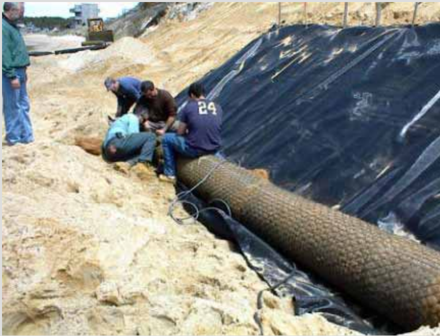
Fiber Roll Installation - Bottom Row
