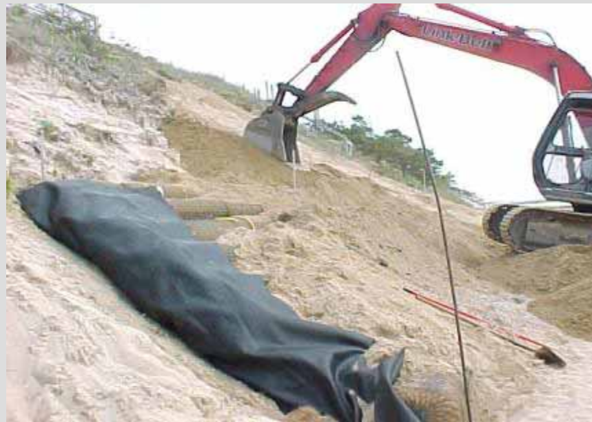
Fiber Roll Installation - Sand Cover
