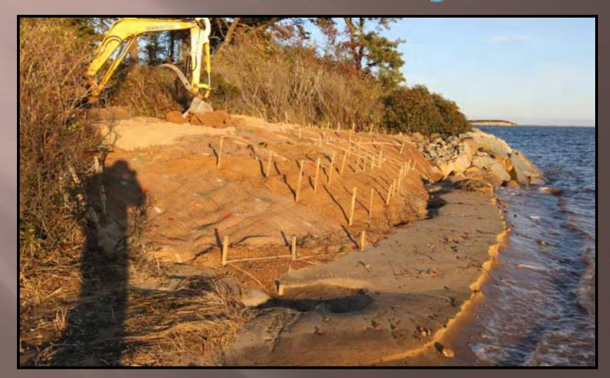
Heavy Coir Erosion Control Blankets to Hold Sediment During Plant Establishment Period
