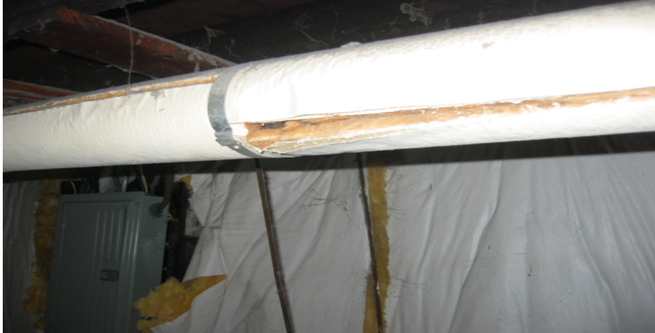
Family Scattered Site 705-1 Development, 7 Maple Street, Basement – Pipe Covered with Exposed Asbestos
