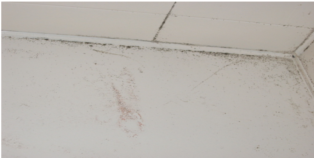
Family Scattered Site 705-1 Development, 7 Maple Street, Bathroom Ceiling Has Black Mold
