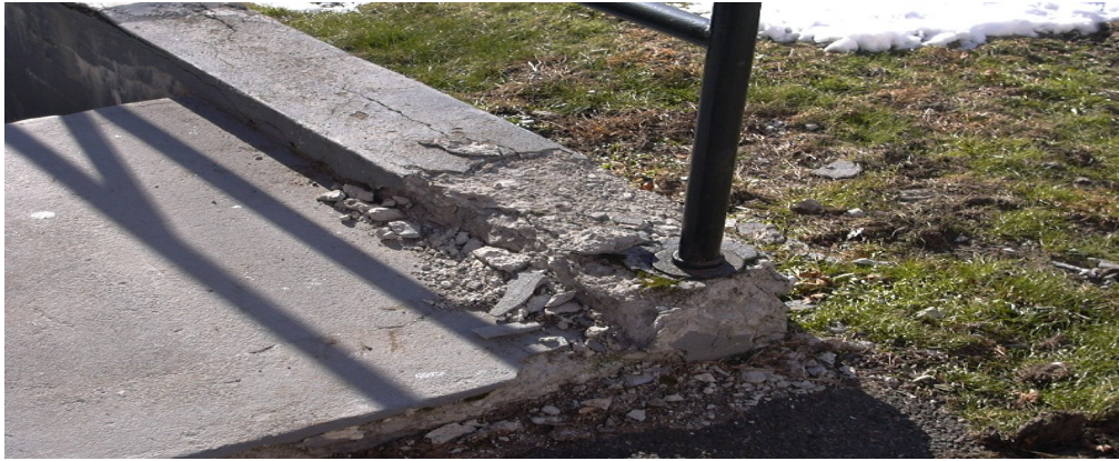
Building Exterior – Cement Railing Support is Crumbling
