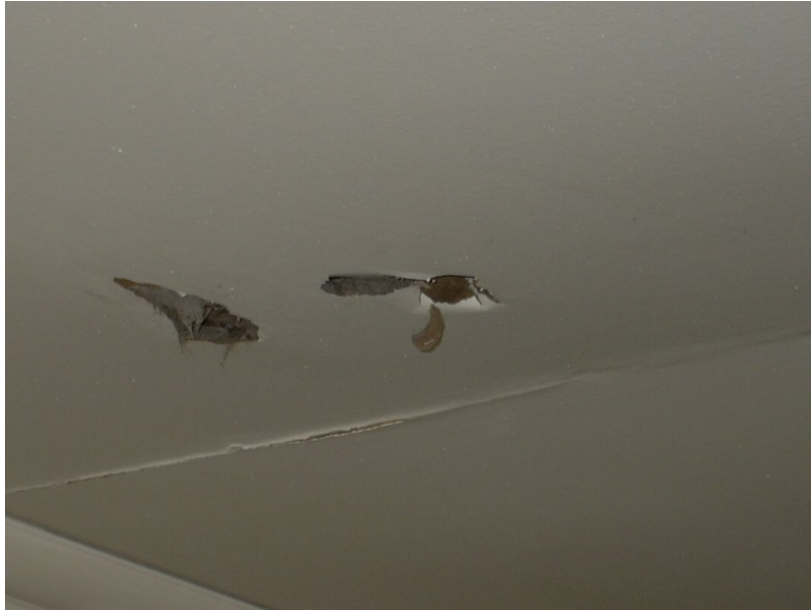
667-C Elderly Housing Development 170 South Common Street, Excessive Water Damage on Ceilings
