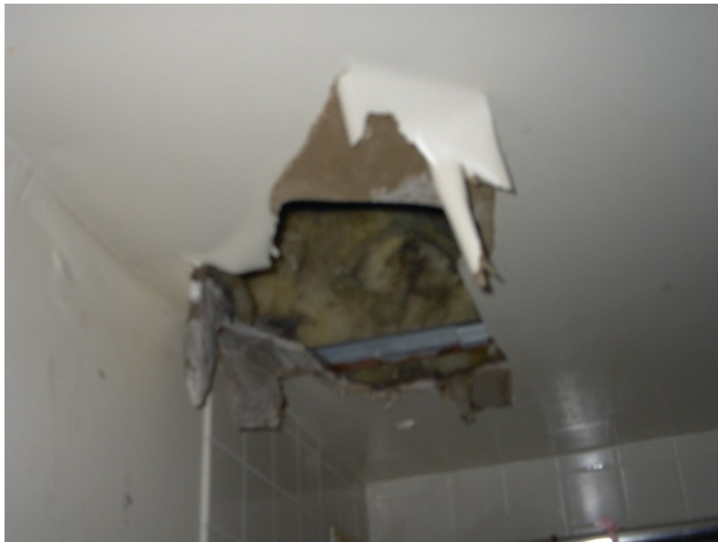
667-C Elderly Housing Development 170 South Common Street, Excessive Water Damage on Ceilings
