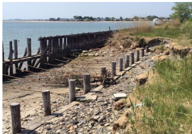
Figure 10. Damaged Seawall near Riley Way, Source: Lynn Coastal Resiliency Assessment, 2016
