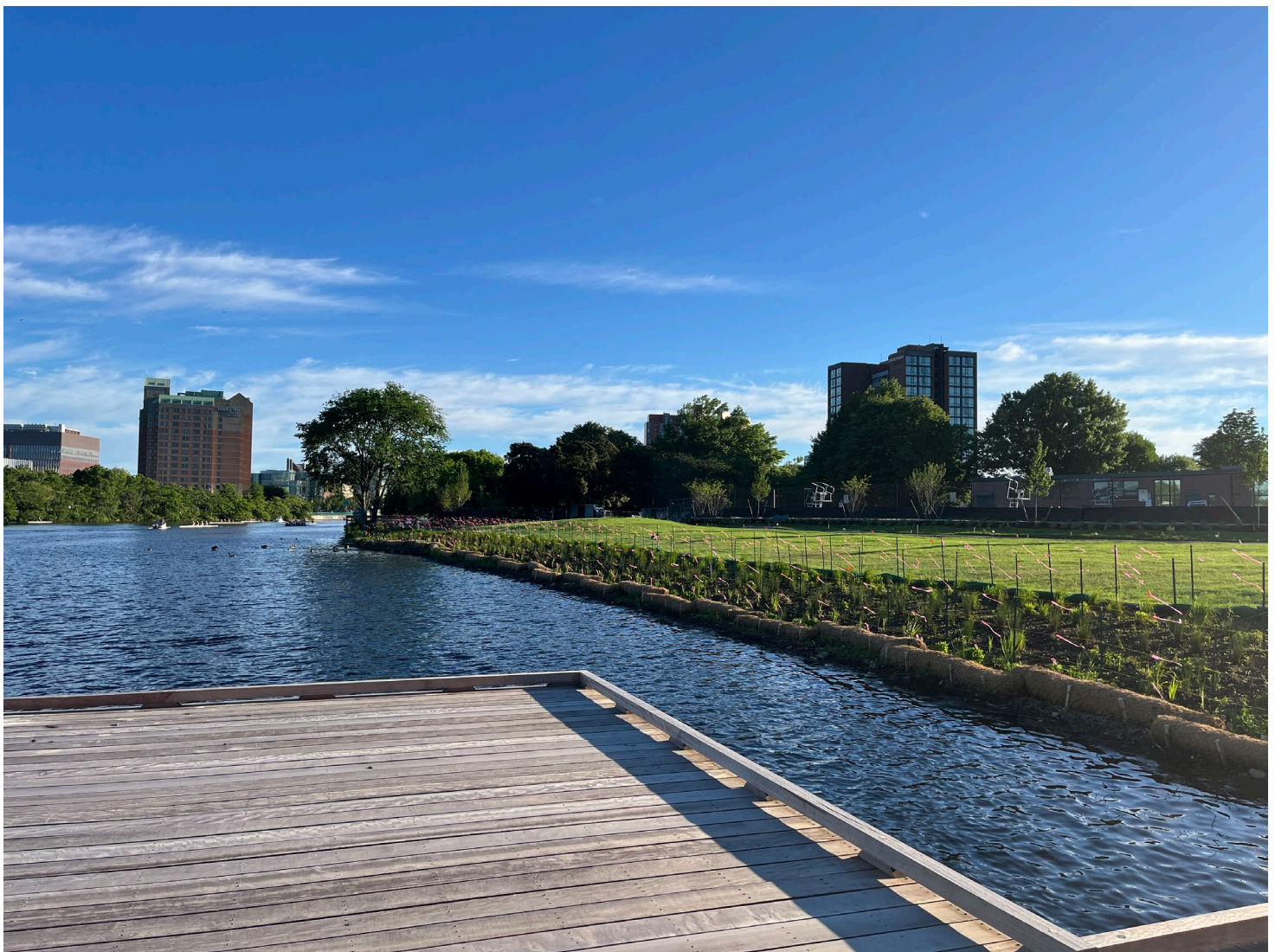
The image above is taken from the new 54' x 18.5' dock looking across the shoreline
