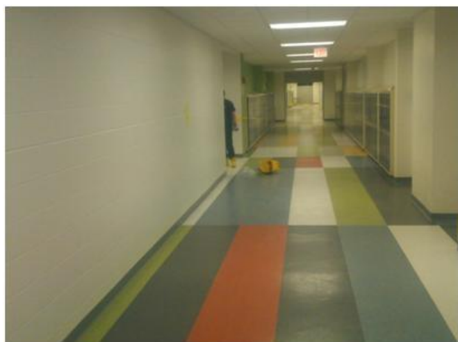
Hallway south of catwalk, looking south
