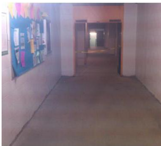
Hallway perpendicular/easterly of Room B-215 hallway, looking north
