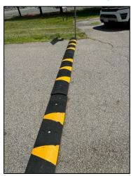
The town reviewed options for temporary speed bumps for the area. Since the area around the train station is being redesigned the measures were selected based on their inexpensive cost and ease of installation. The temporary bumps are typically installed after the last plowable snow in the spring and removed before the first plowable snow in the winter.
