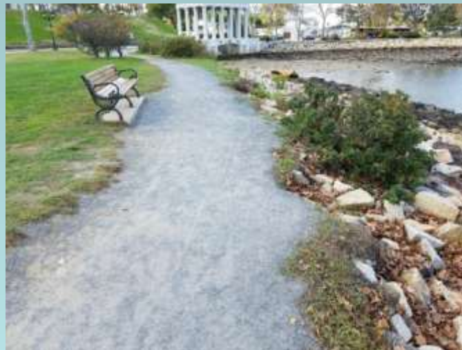
Localized collapses along rip rap
