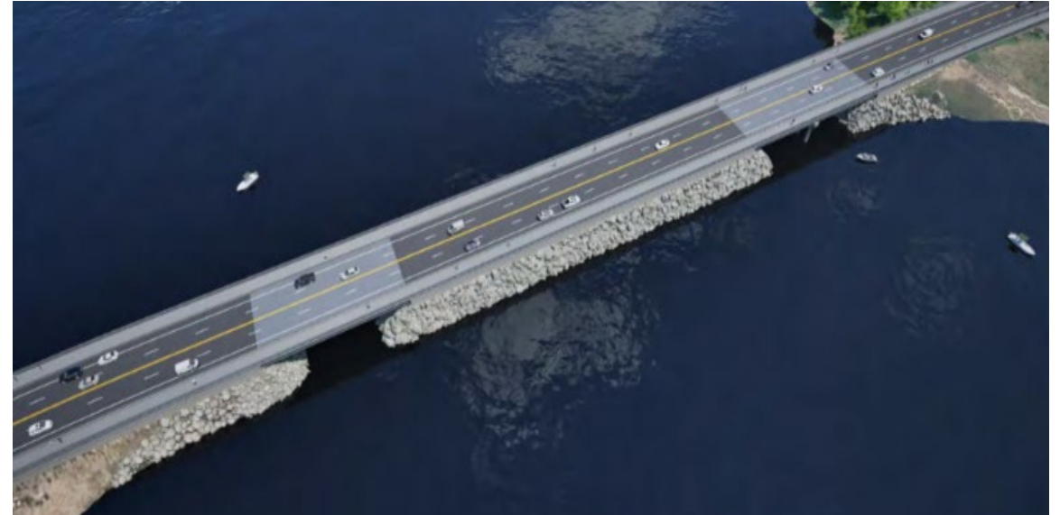
Marion/Wareham Road over Weweantic River
