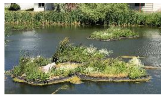
Floating islands in a stormwater pond (courtesy of Floating Island International)
