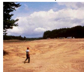
Dry dredging of Dunn's Pond in Gardner with conventional excavation equipment (above) to a “hard” bottom (below) (provided by C. Carranza of BEC)
