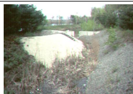
Filter berm acting as outlet for a detention area
