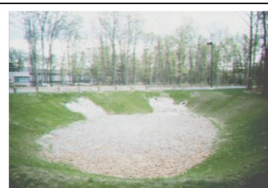
Combination detention and leaching basin
