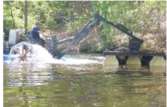
Hydrorake placing raked material on a push barge for offloading at a designated site
