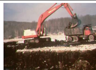
Dry dredging of Dunn's Pond in Gardner with conventional excavation equipment (above) to a “hard” bottom (below) (provided by C. Carranza of BEC)
