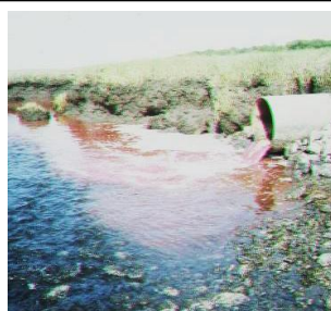
Wastewater point source discharge
