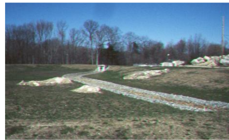
Infiltration trench
