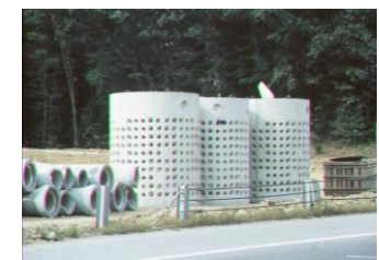
Leaching catch basin vaults
