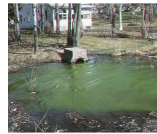
Stormwater point source discharge
