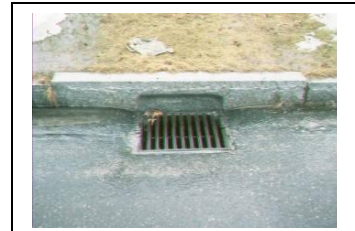
Drainage inlets typically lead to pipes that become stormwater point source discharges
