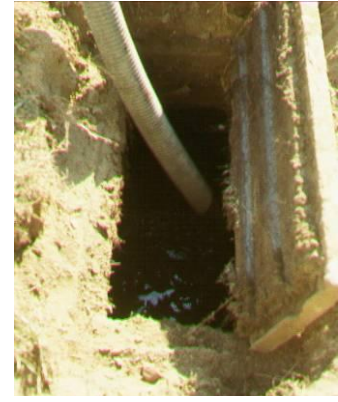
Septic system pump-out
