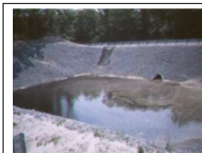
Wet detention basin
