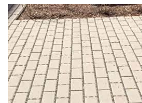
Porous Pavement (Source: USEPA)
