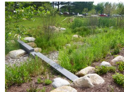
Small bioretention area/rain garden (above) and larger, more elaborate area (below)
