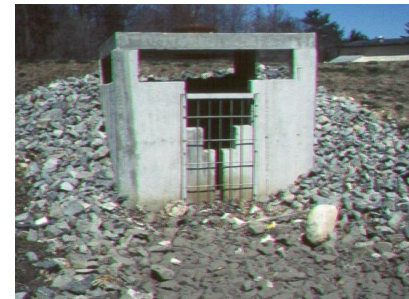
Dry detention basin (above) and flow control outlet (below)
