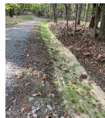
Newly established swale with stabilization mesh supporting vegetation growth
