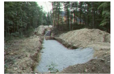
Septic system leachfield being installed
