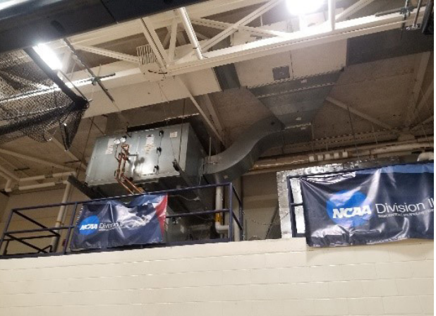
Elevated Location for Mechanical Equipment
