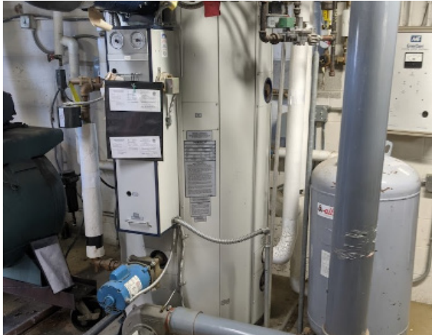
Condensing Gas Fired Domestic Hot Water Heater
