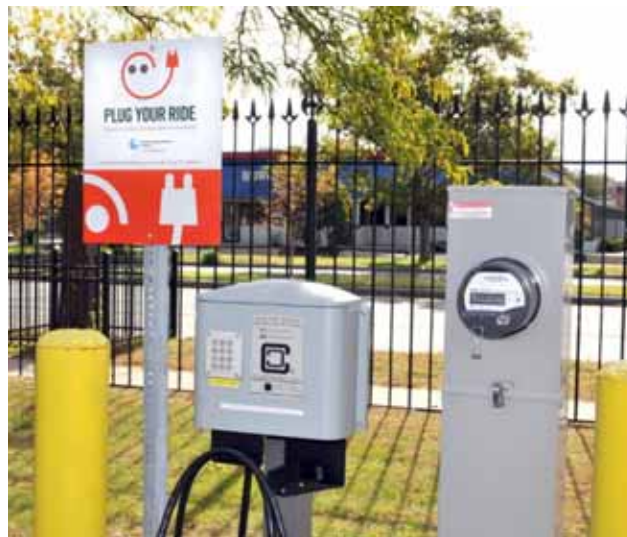
Figure 20. Eversource ClipperCreek EVSE.
