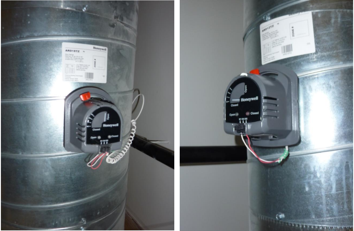
Photo 3 – Zone Dampers in Fully Open and Fully Closed Positions
