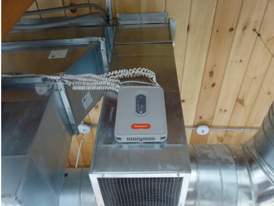
Photo 4 – Bypass VAV System Controller
