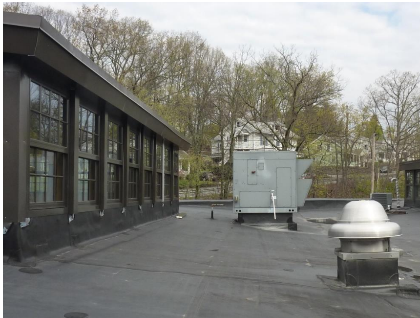
Photo 1 – Representative Rooftop Unit (RTU-1, note gas supply not connected)
