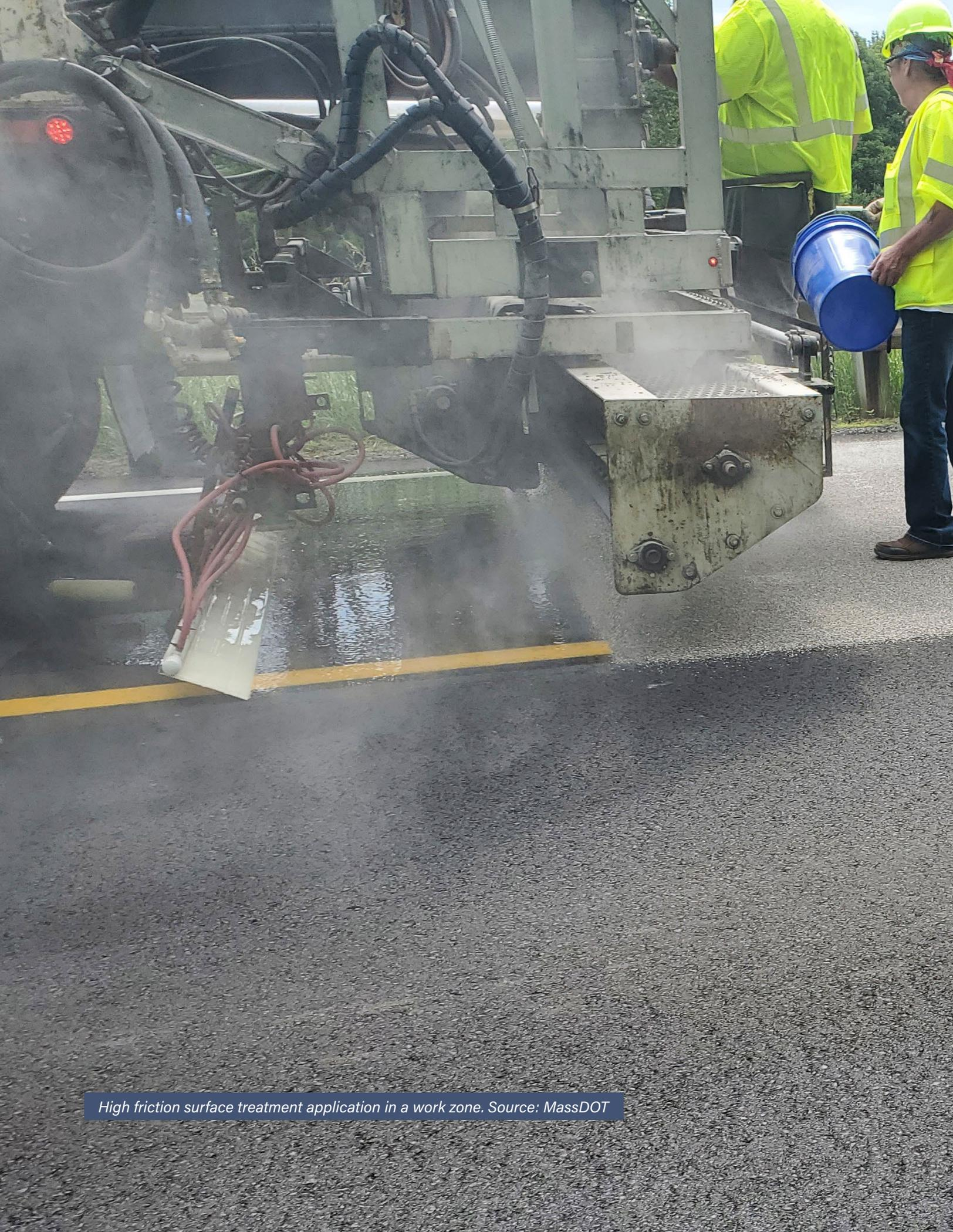
*High friction surface treatment application in a work zone. Source: MassDOT*
