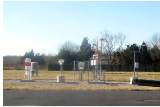
AWOS System (Marshfield Municipal Airport)
