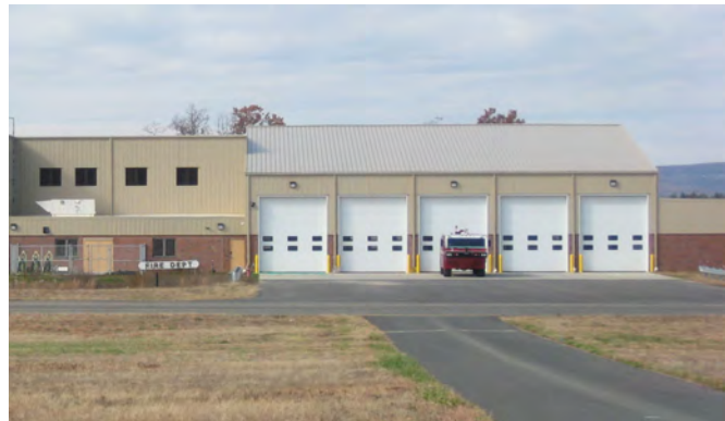
ARFF Facility (Barnes Municipal Airport)
