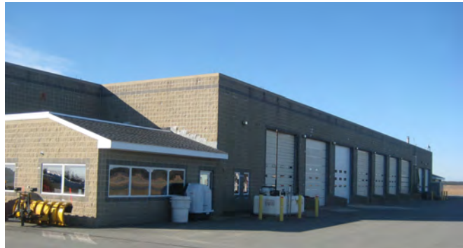
Snow Removal Equipment Building (Barnstable Municipal Airport)
