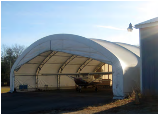
Portable Hangar (Sterling Airport)
