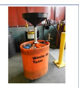
This waste oil caddy can be wheeled over to an oil collection tank and drained directly into the tank using an air supply.
