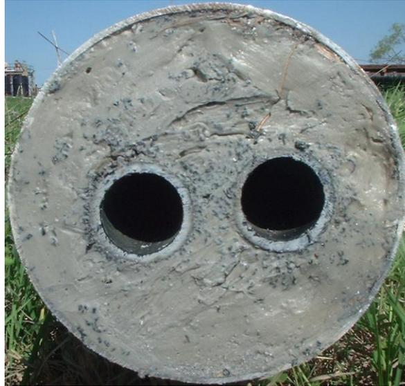
1. Grouting with Tremie under pressure from bottom to top.
