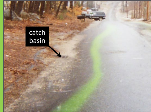
Dye test showing stormwater bypassing the intended flow path to a catch basin.
