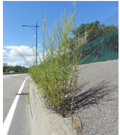
Photo 1 – Mugwort in difficult to access median blocks sight distances and leads to structural degradation.
