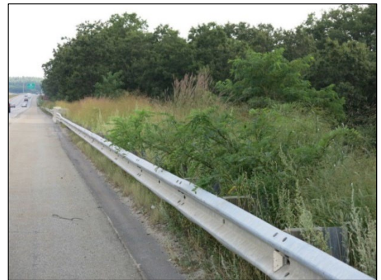
Photo 5- Switchgrass behind guardrail in this location does not require management as it does not pose a safety concern. Targeted herbicide treatment could be used to eradicate problematic plants such as black locust.
