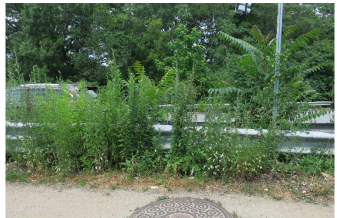
Photo 2 – Rapid re-growth or re-sprouting of mugwort and tree of heaven in median guardrail creates visibility and structural problems and is unsightly.
