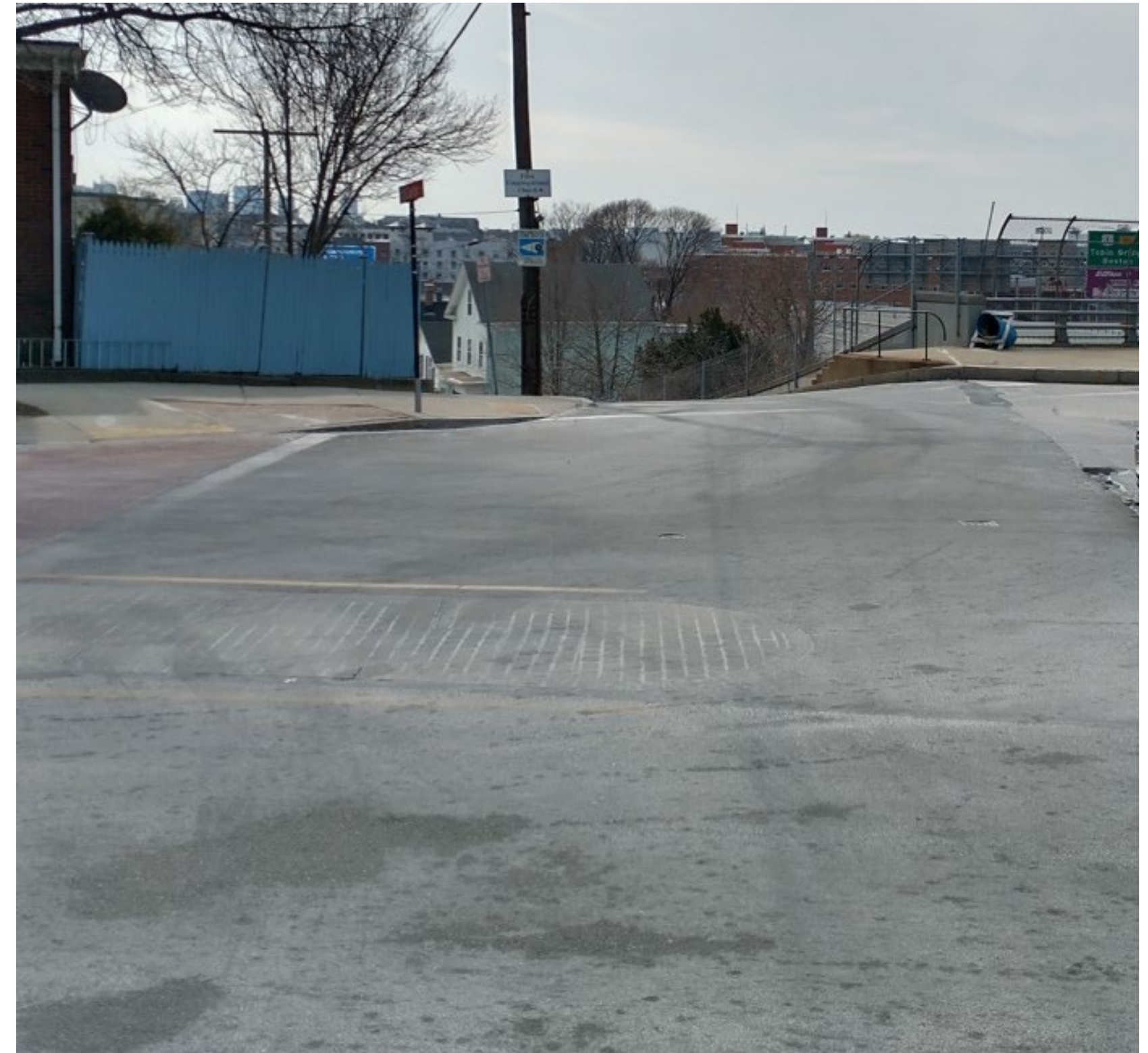
Deck has numerous patches and areas of deterioration
