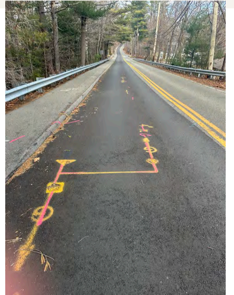
Existing Guardrail on Merriam Street
