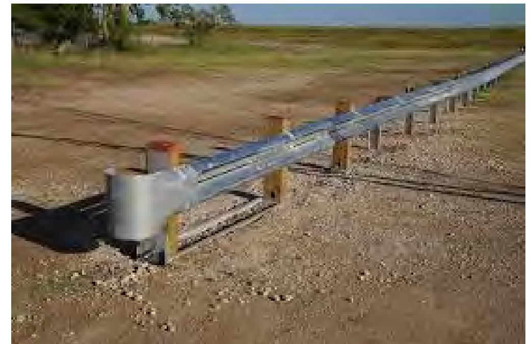
MASH TL-2 W-Beam Guardrail
