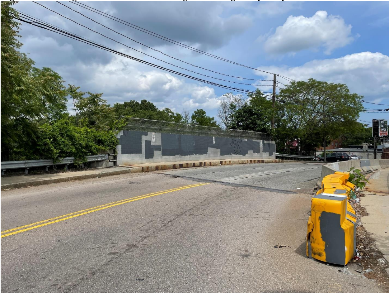
Figure 2: Existing Conditions On The Bridge Including Temporary Barrier
