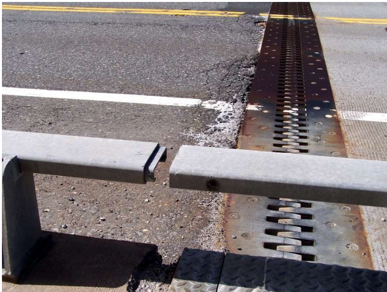
Potential Snag Point at Expansion Joint
