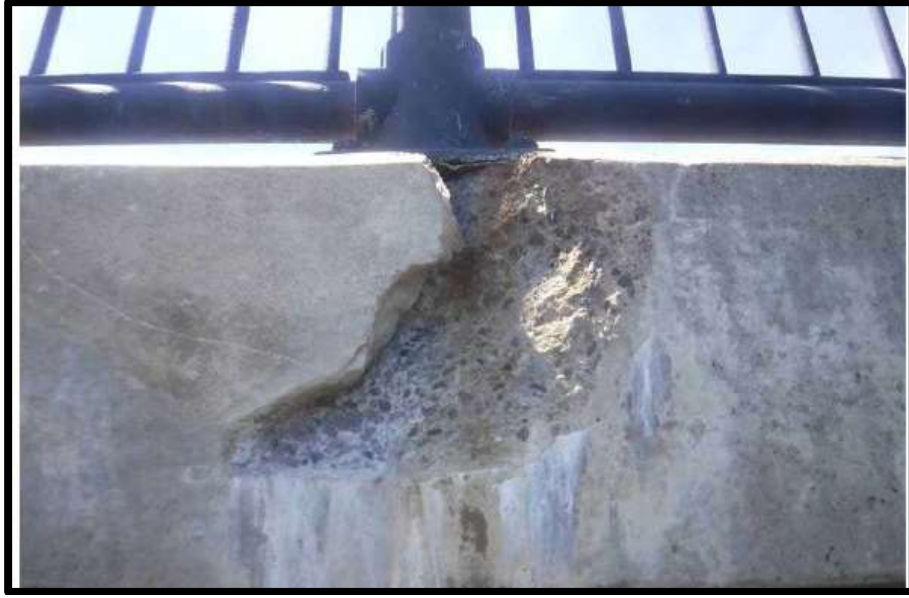
Spalling Concrete at Copings
