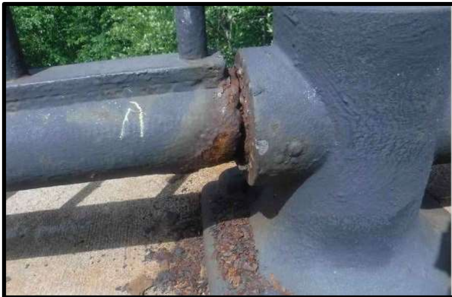
Deterioration at Pedestrian Rail
