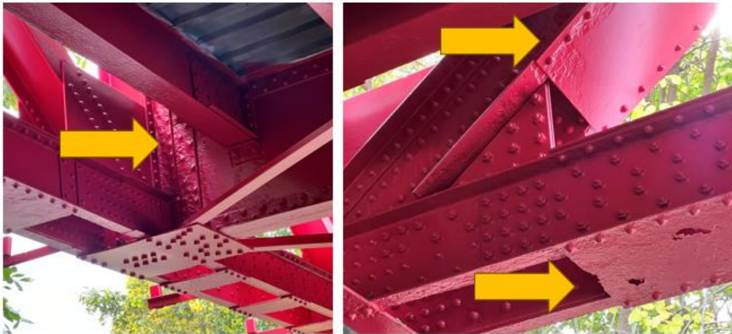
Figure 3: Recent Cleaning and Painting Hides Critical Section Loss
