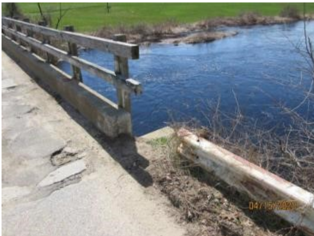
Image 10 – Northwest approach guardrail low to the ground and not attached to bridge rail
