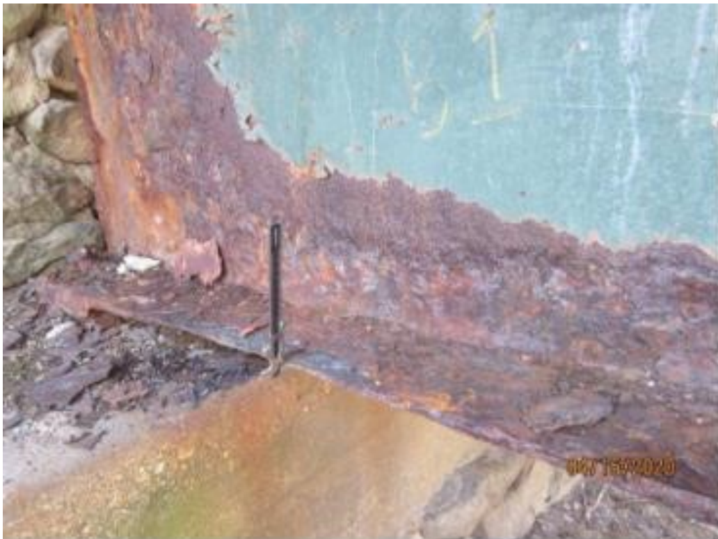
Image 8 – East face of deteriorated East Girder at South Abutment
