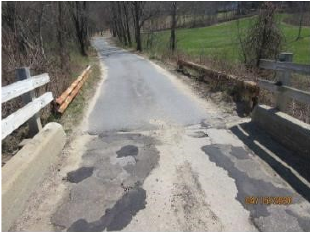
Image 9 – Severe deterioration at south end of deck surface
