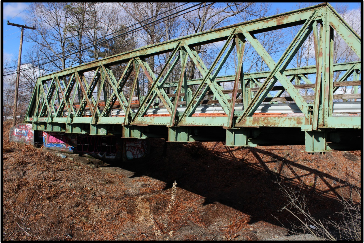
Existing West Elevation View of Bridge
