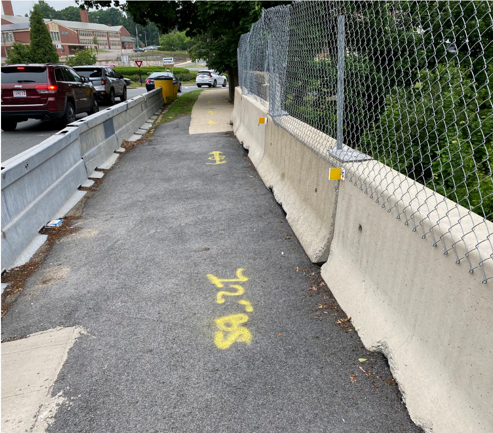
Temporary Traffic Barriers in place along roadway and railing
