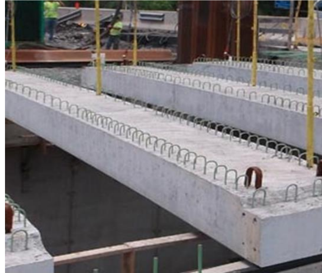
Prestressed Concrete Box Beam
