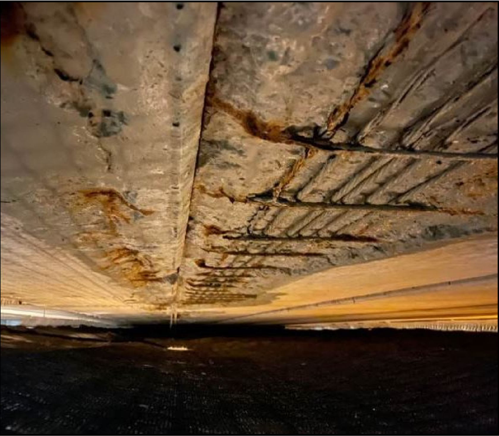
Deterioration to existing beams
