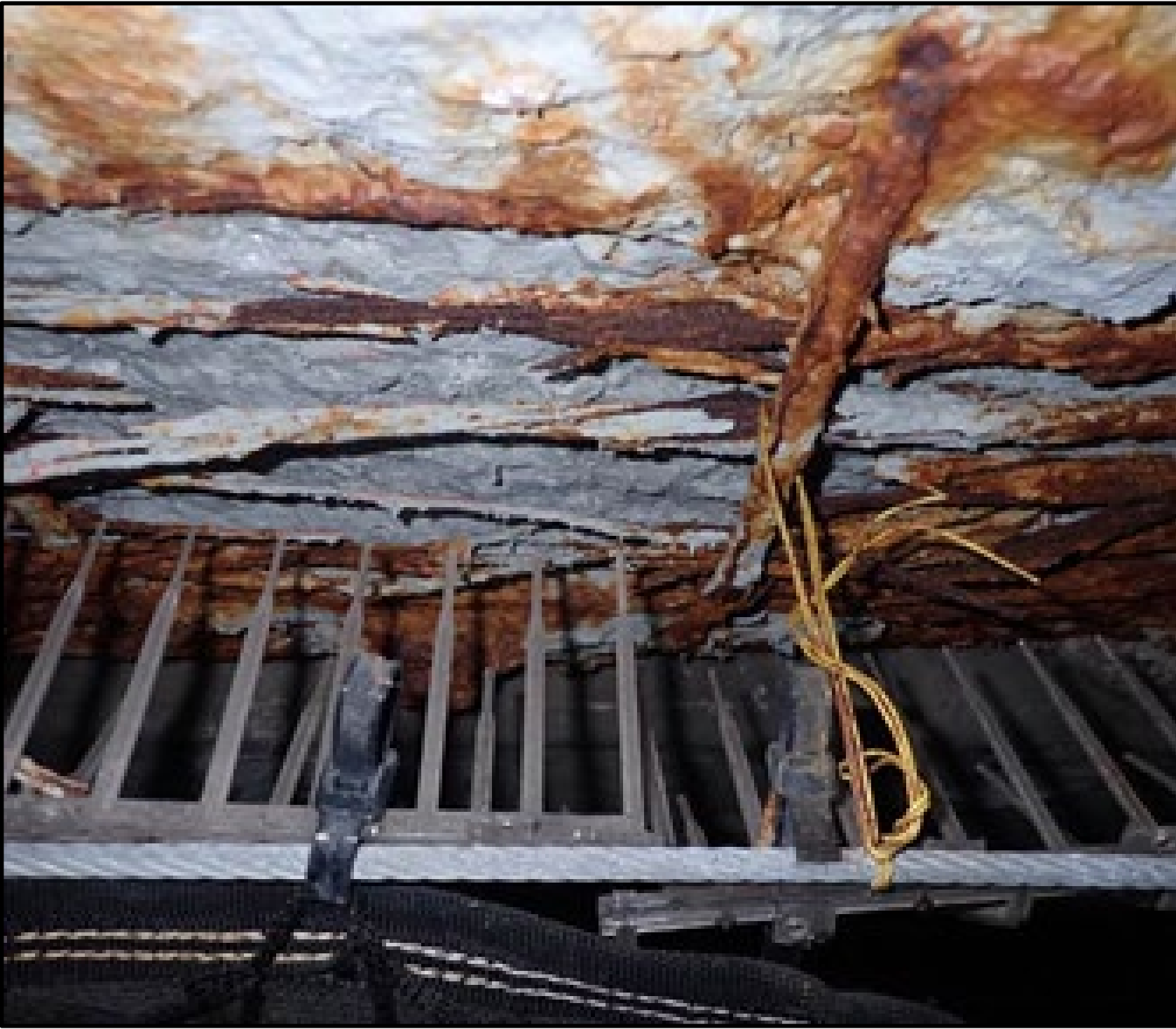
Deterioration to existing beams
