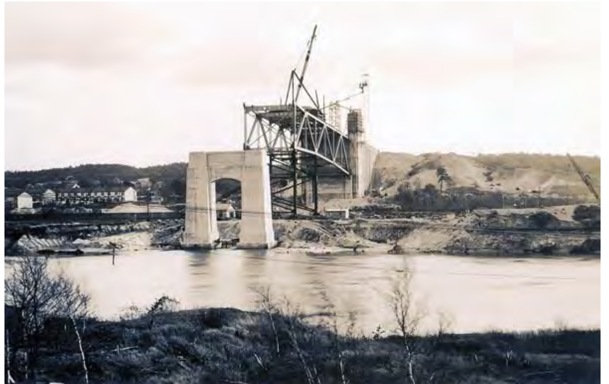
Sagamore Bridge Construction circa 1934
