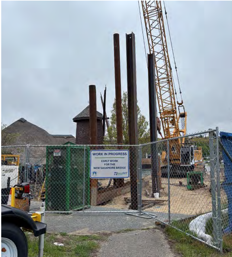
Driven Piles – Location #1
