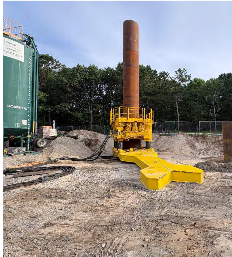
Drilled Shaft – Location #3
