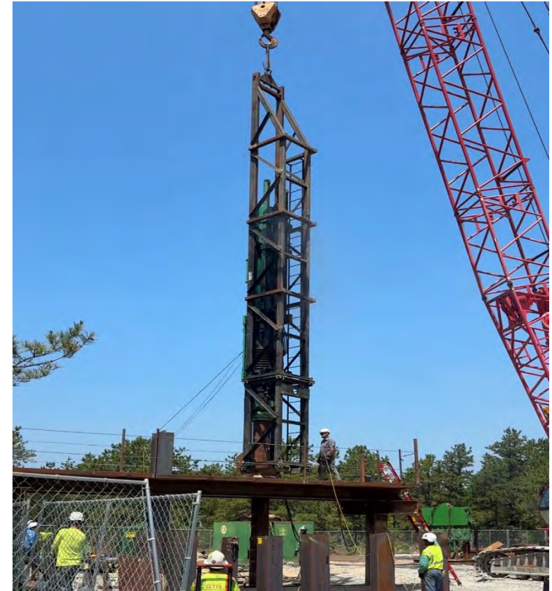
Driven Pile – Location #4
