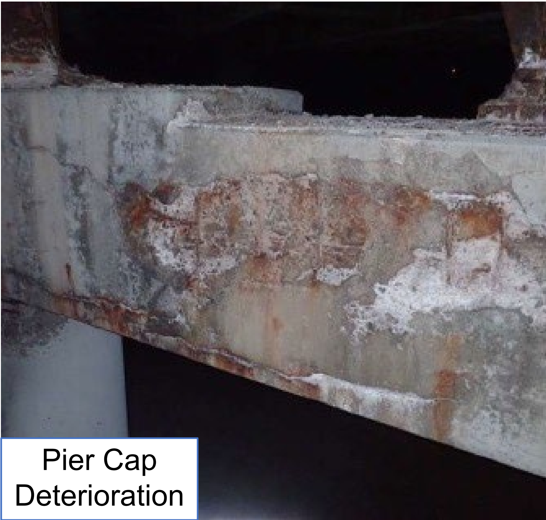
Pier Column Severe Deterioration
