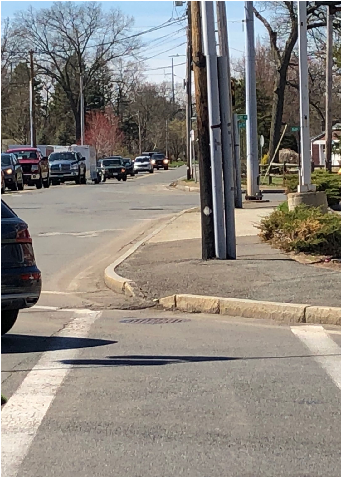
Crosswalks and sidewalk not ADA compliant
