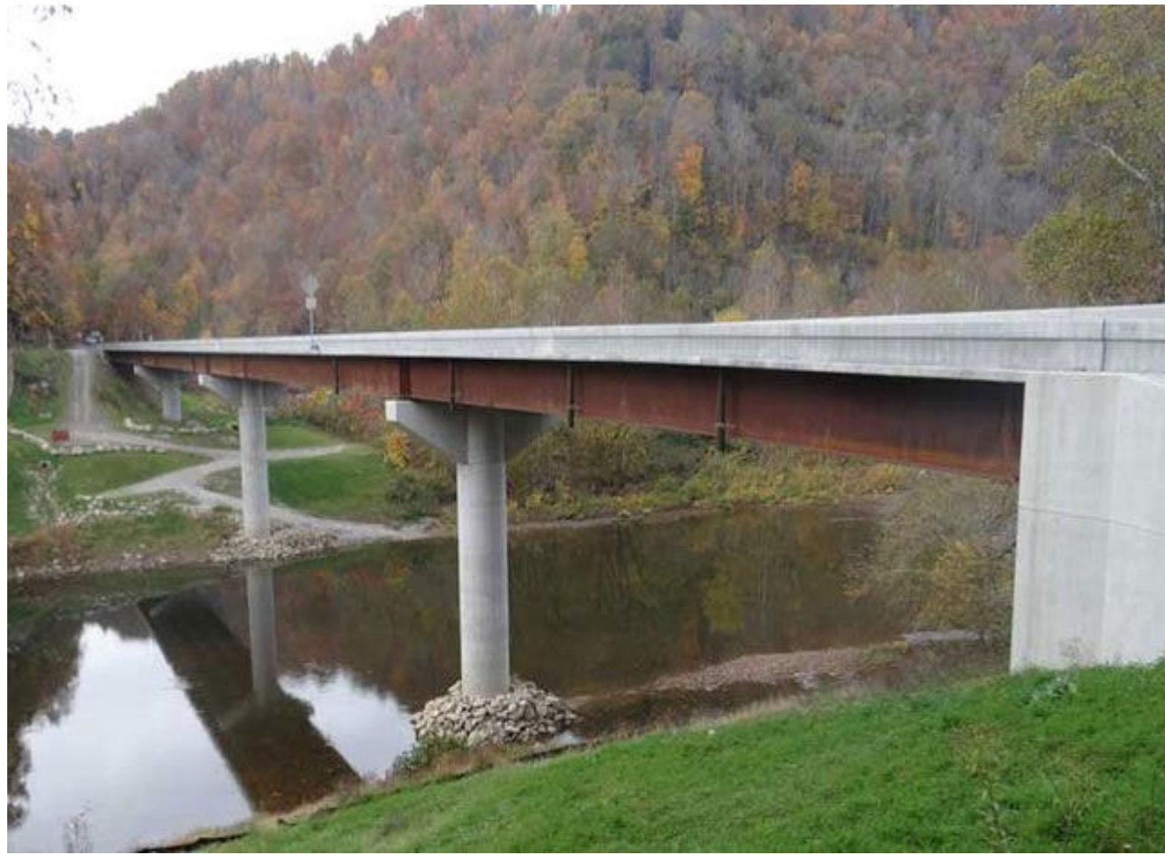
Welded Steel Plate Girder
