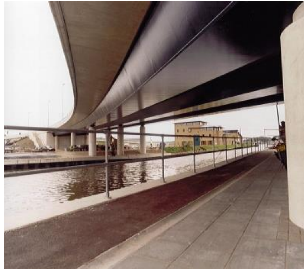
Welded Steel Box Girder
