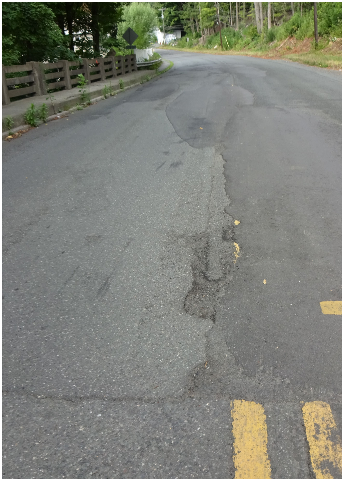
Deteriorated Pavement
