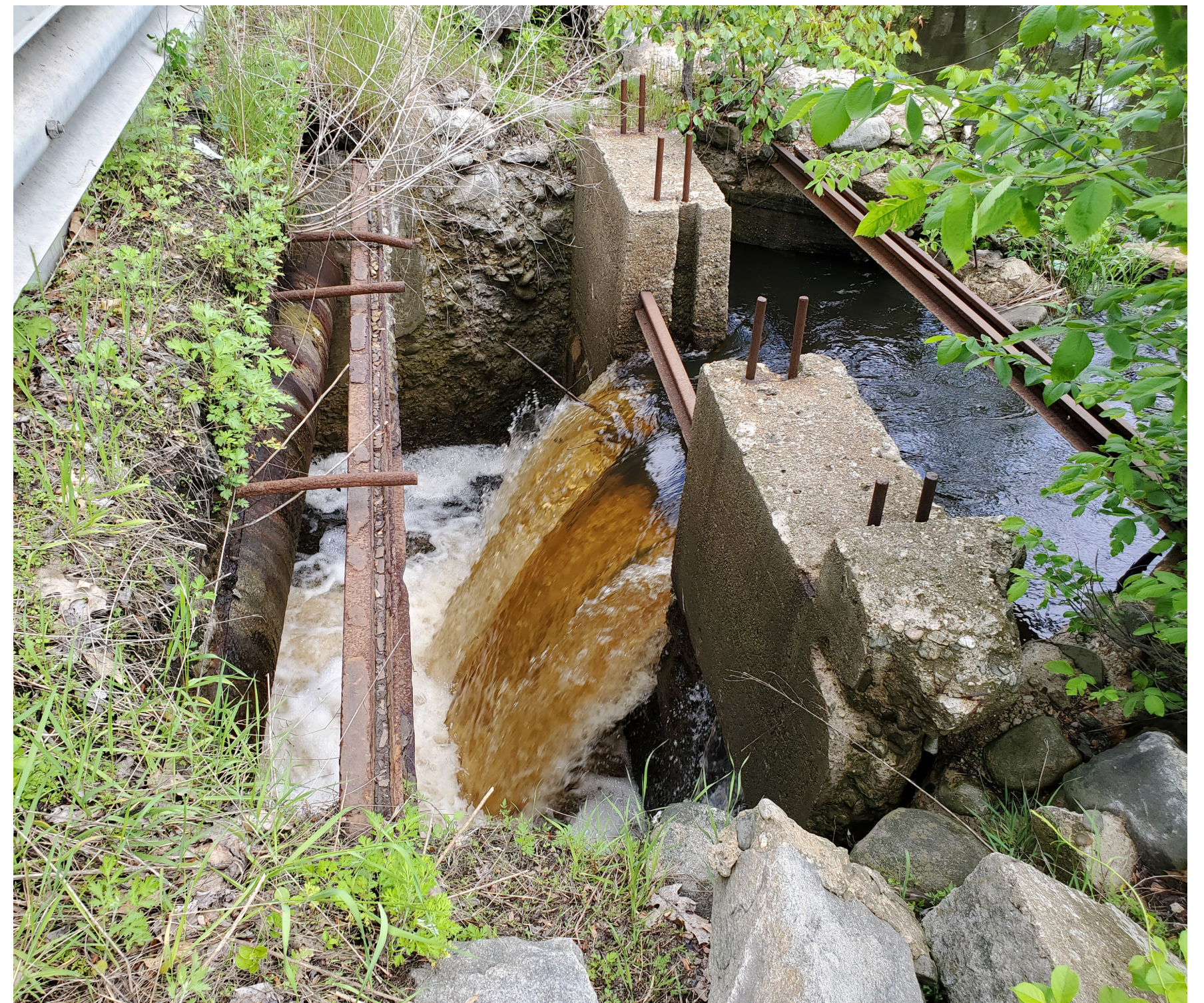
Structurally deficient dam
