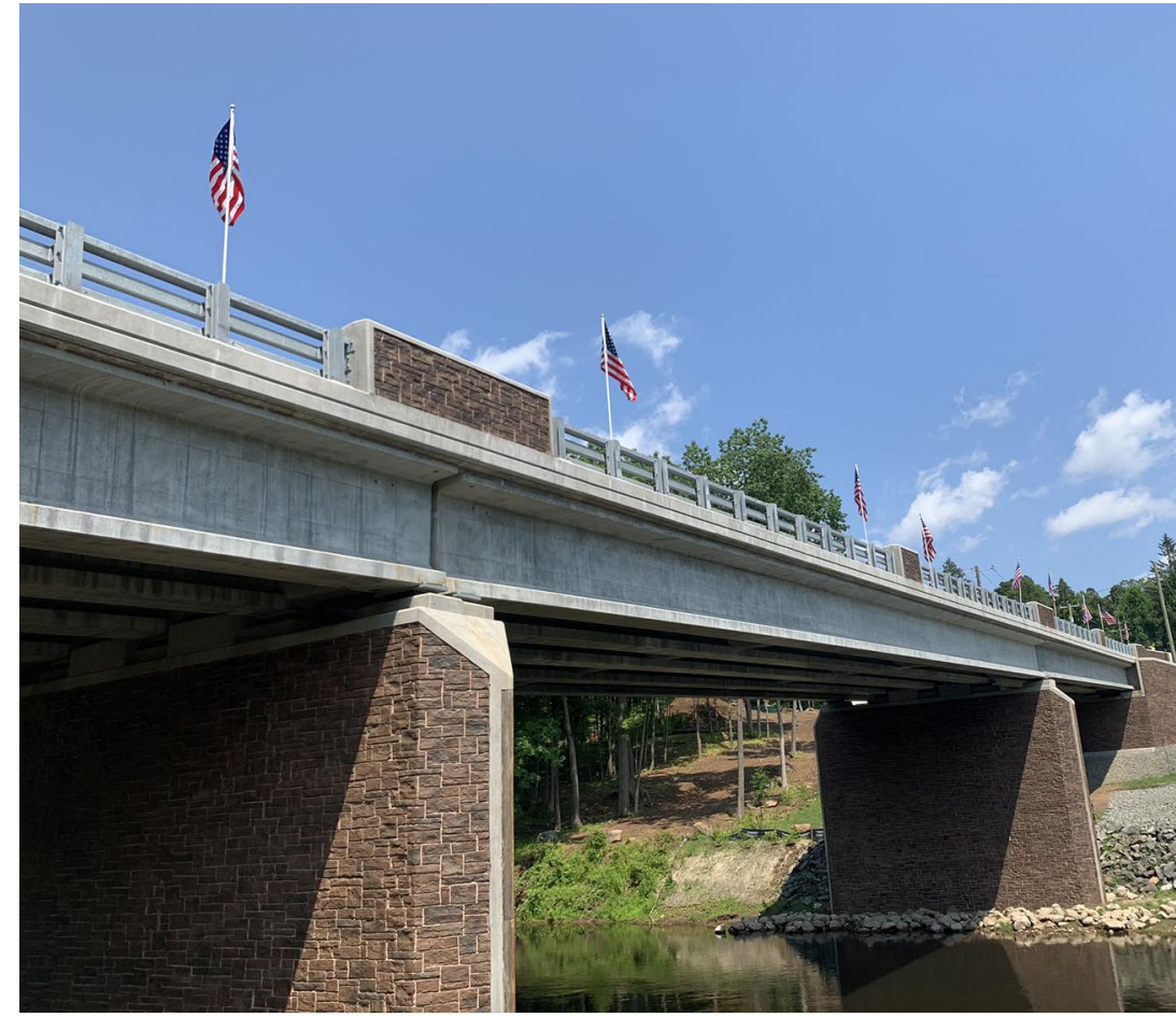
Prestressed New England Bulb Tee Beam
