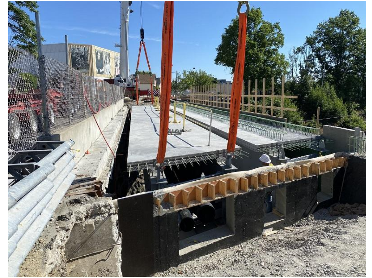
Prefabricated Bridge Unit (PBU)
