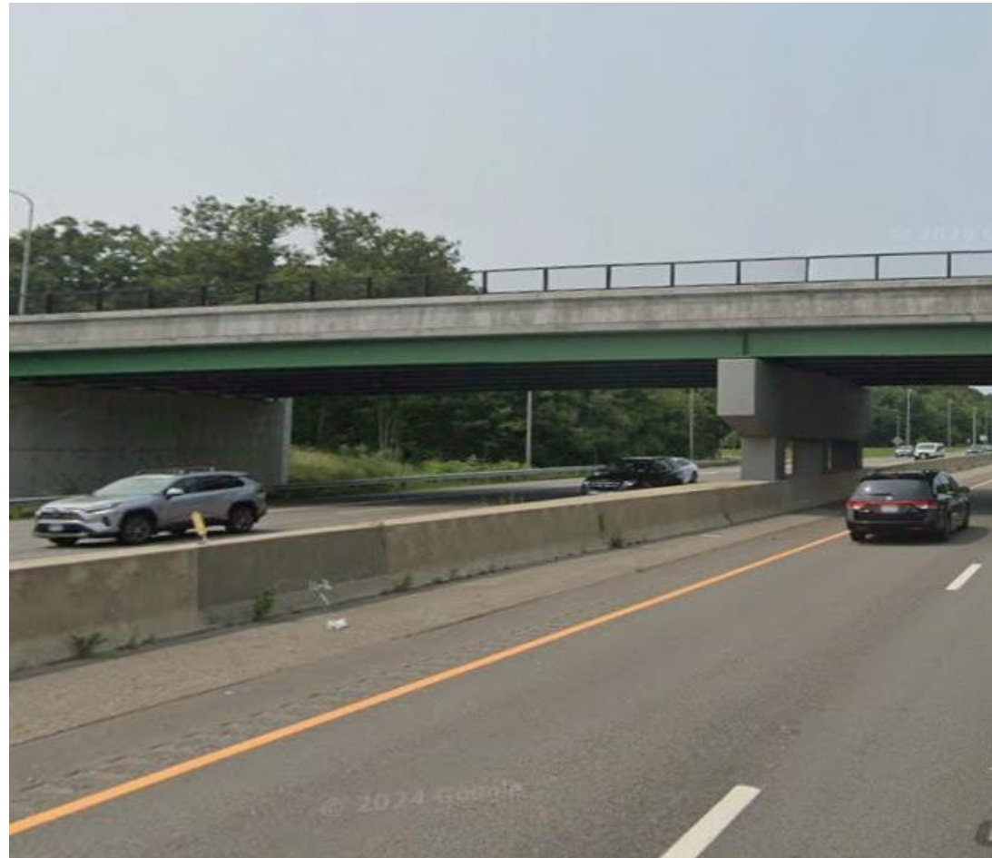
Continuous Steel Plate Girder
