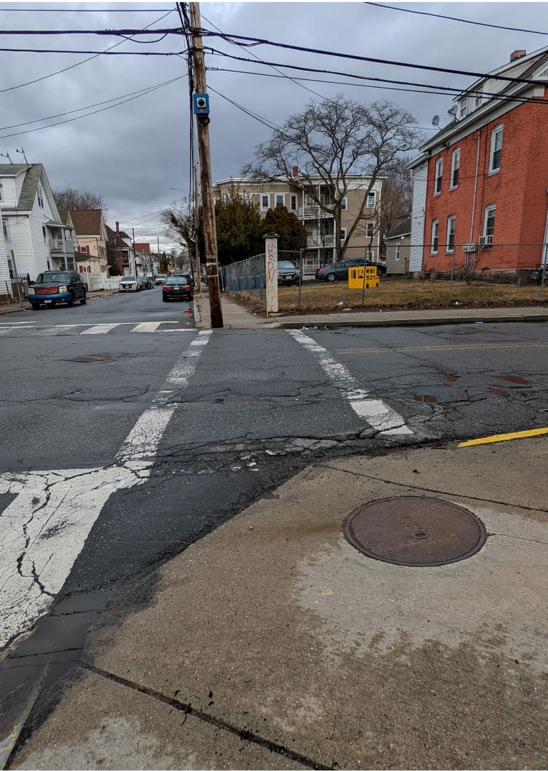
Lack of ADA-compliant pedestrian curb ramps
