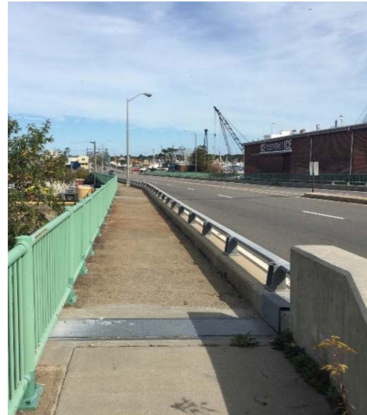
Looking east at sideway on Route 6 Westbound approaching stairway
