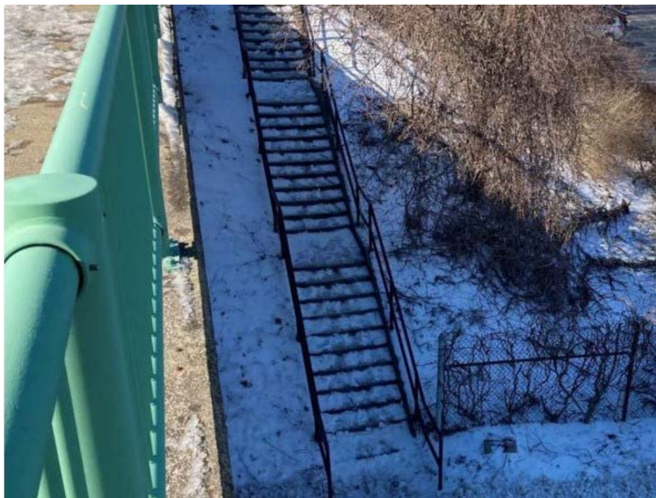
Looking down at existing stairway from Route 6
