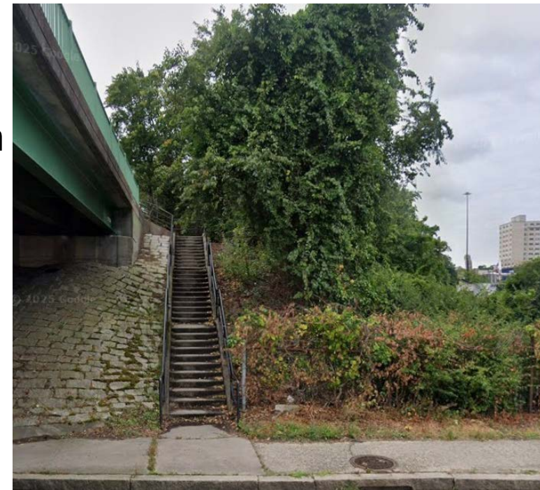
Looking west at existing stairway
