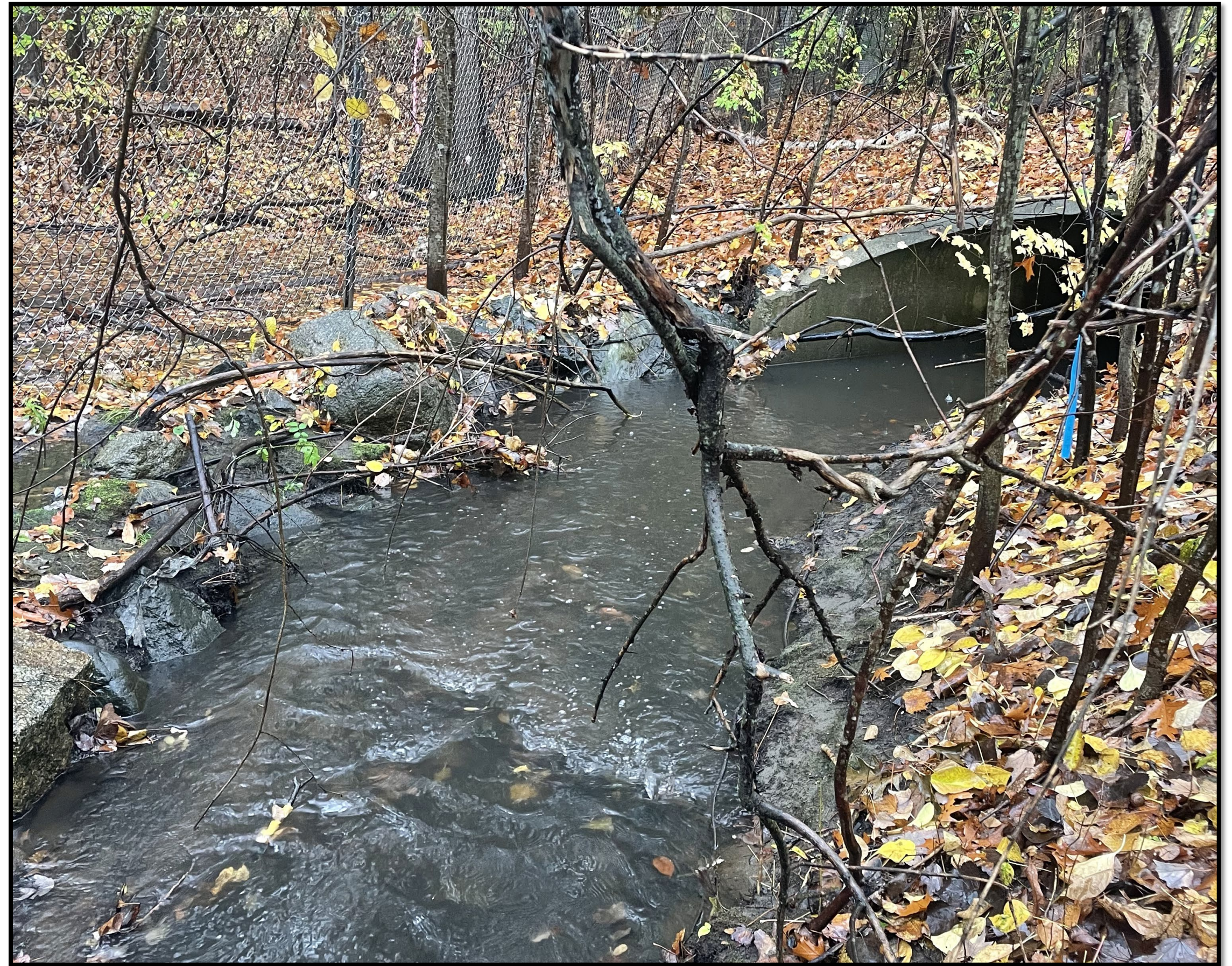
I-95 drainage outfall at the bottom of the embankment
