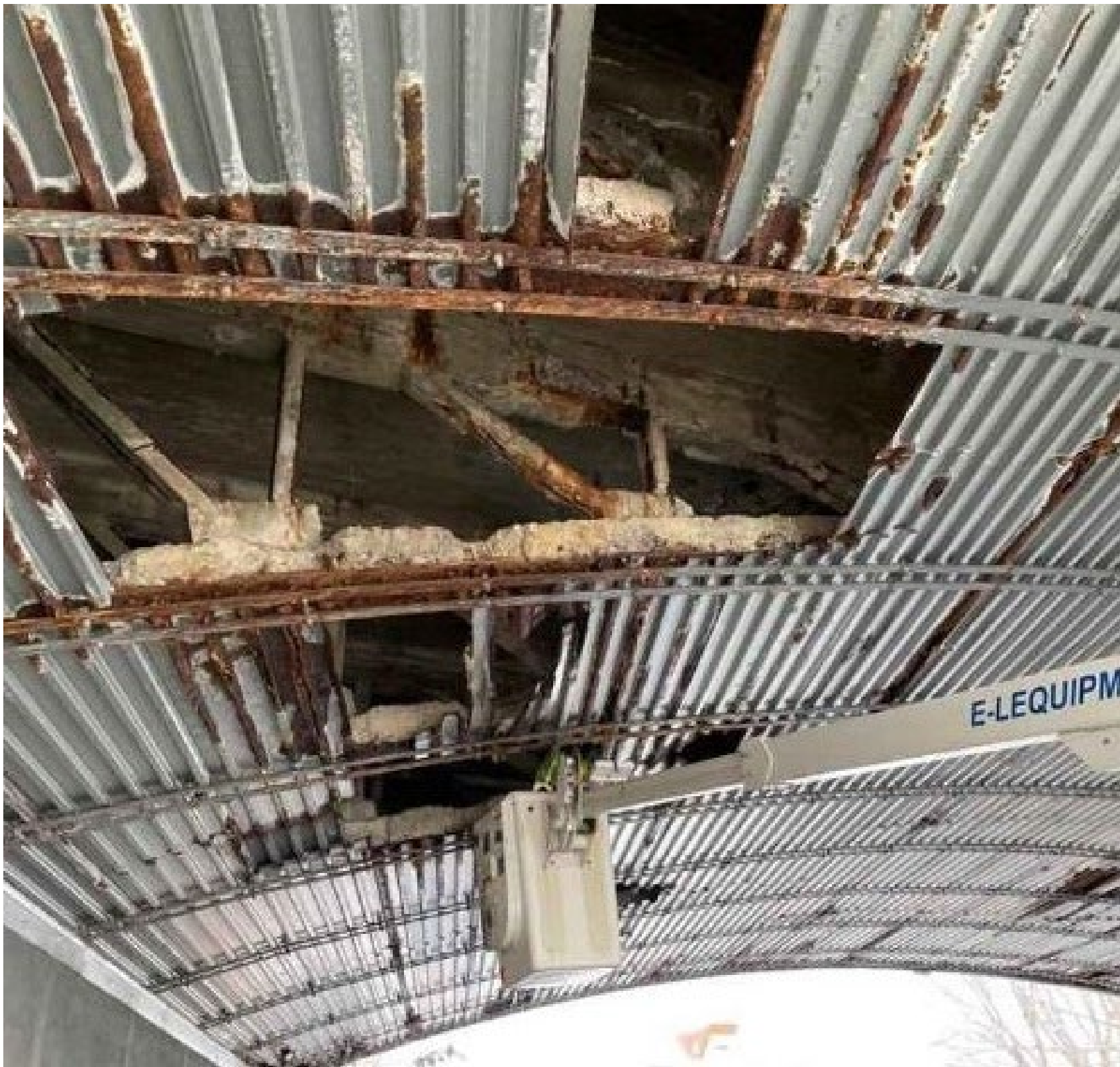
Superstructure frame concrete and steel deterioration
