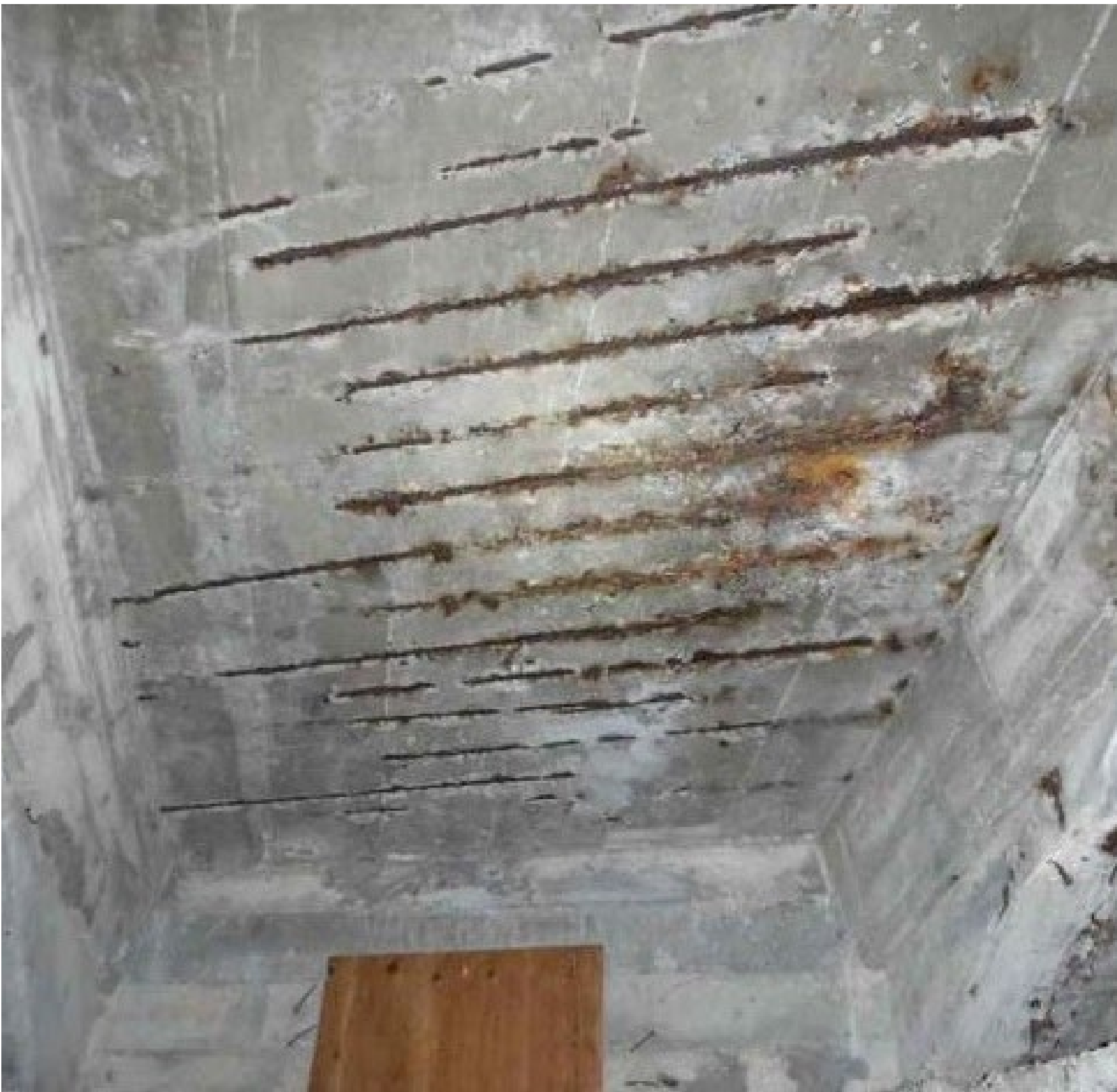
Deck Underside with exposed and deteriorated rebar
