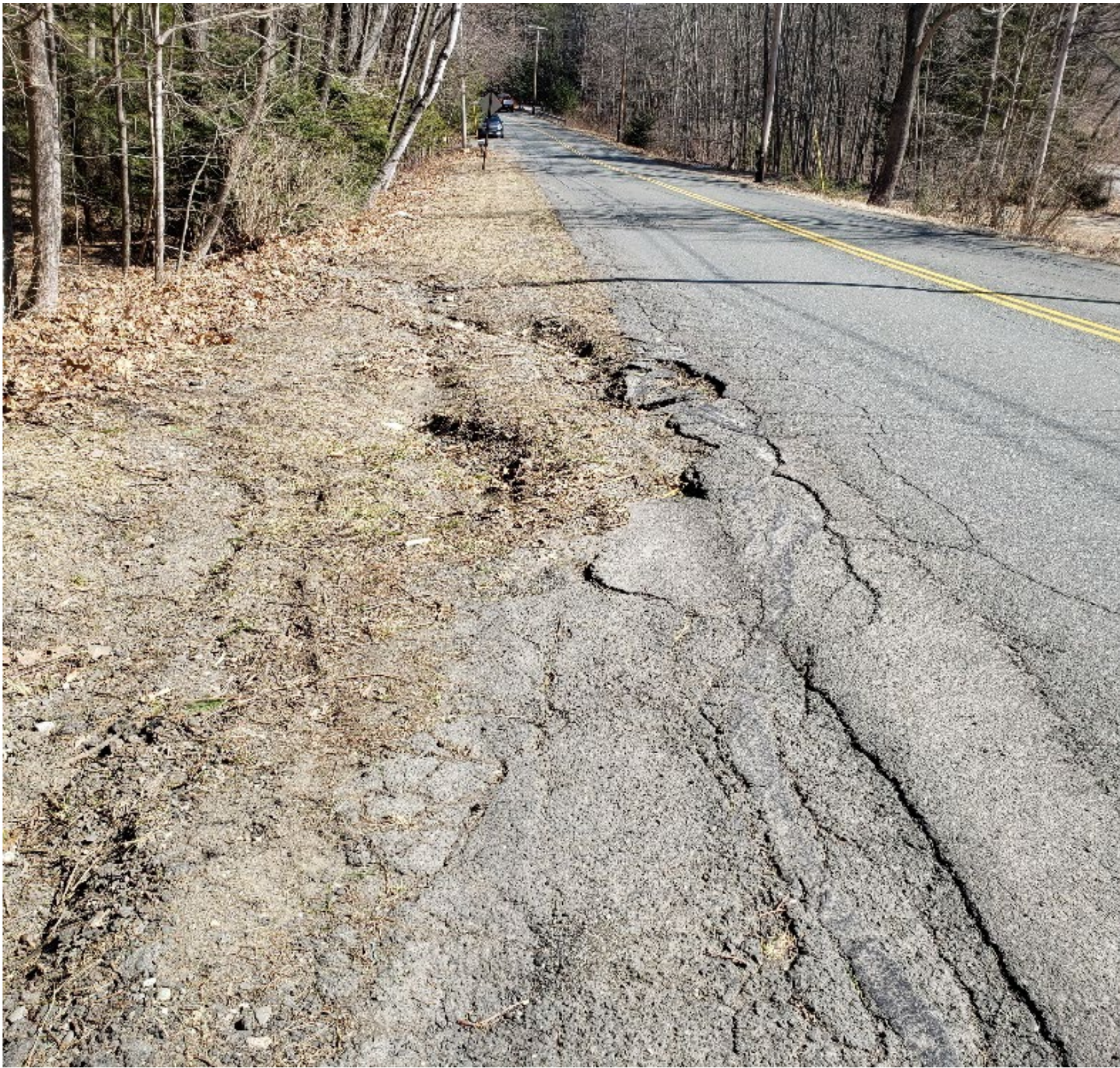
Cracking of the pavement edge and erosion along the gravel shoulder.
