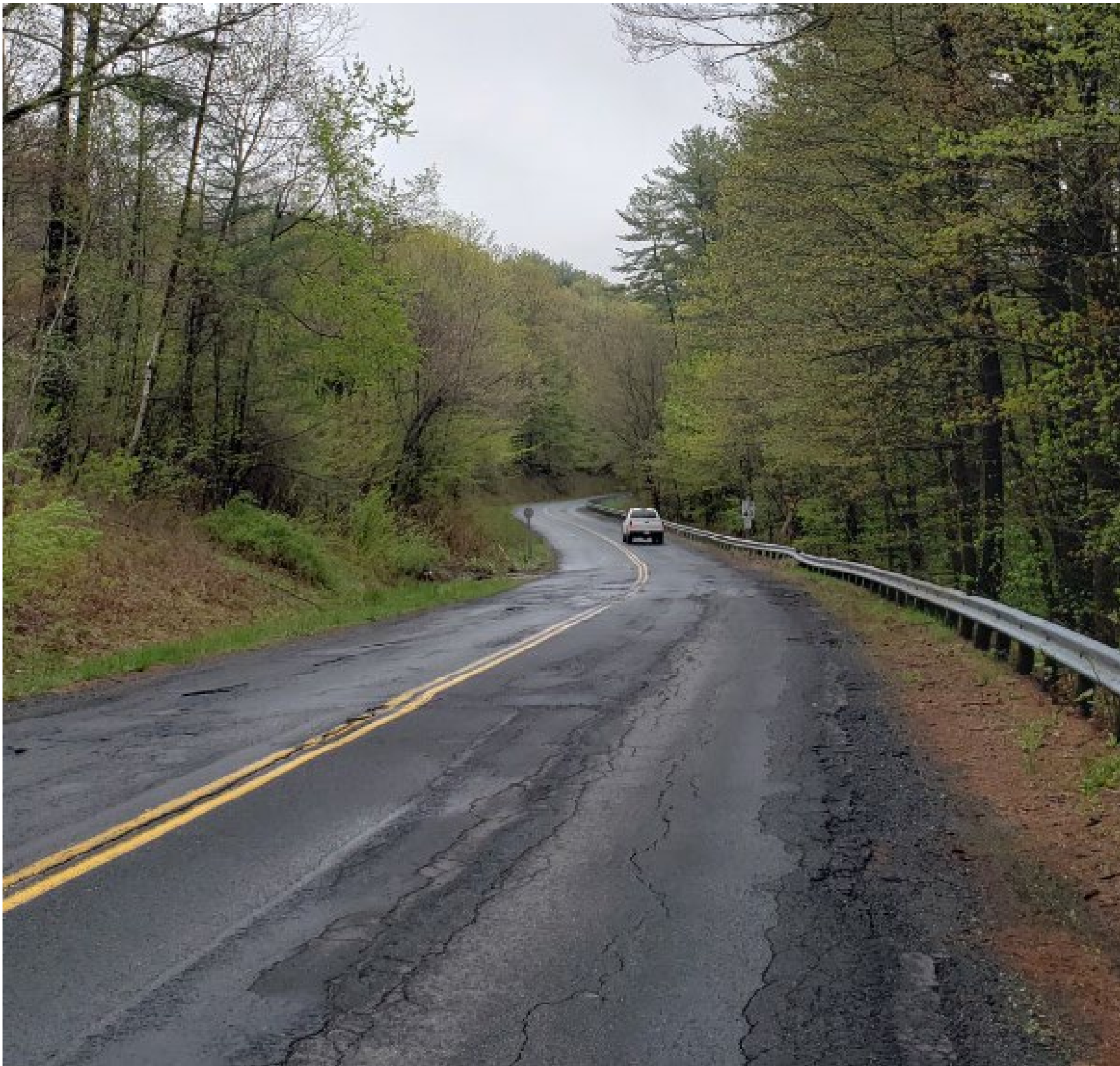
Station 159+20 Roadway pavement is rutting, cracking and fragmenting. Steep back-slope and tree cover
