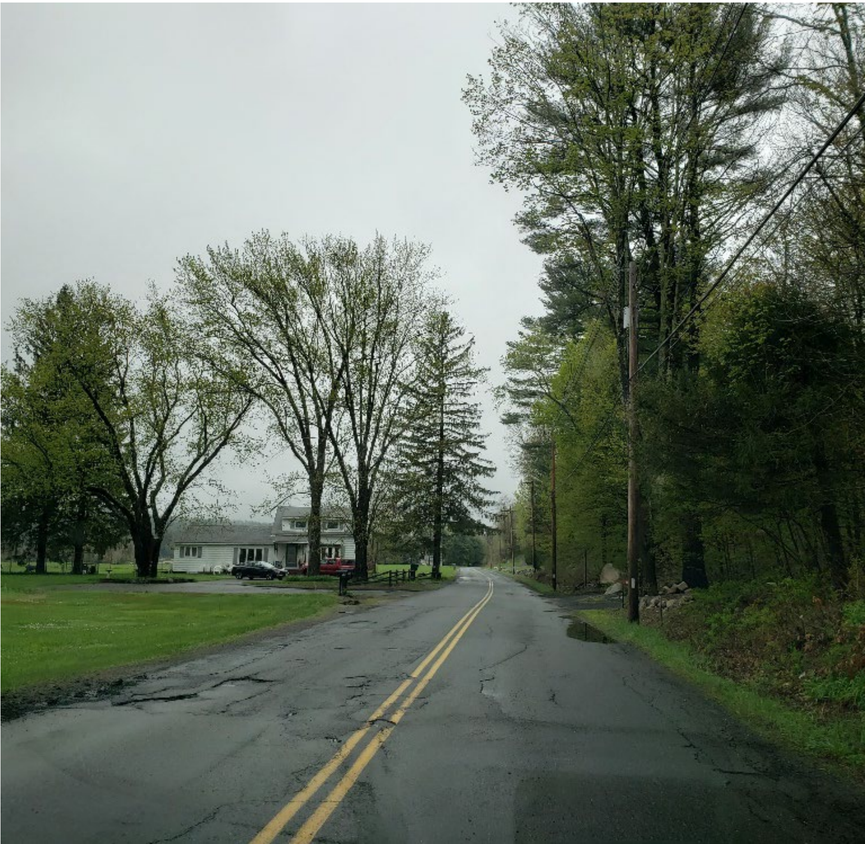
Station 73+50 Ponding at edge of the road, cracking and delaminating the pavement with near-by trees & utility poles
