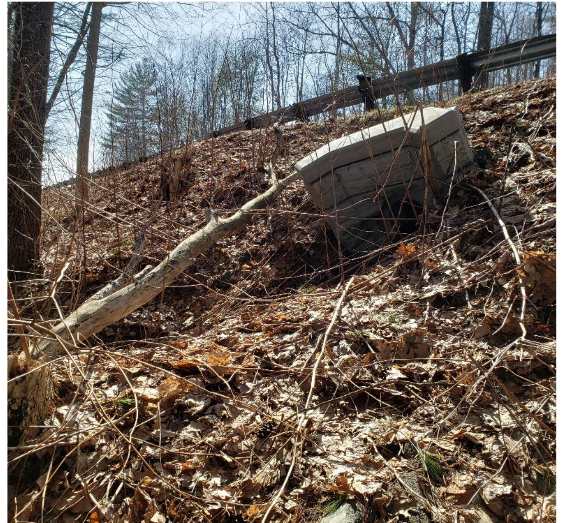
Steep outlet of an existing outfall and the headwall that is falling over.
