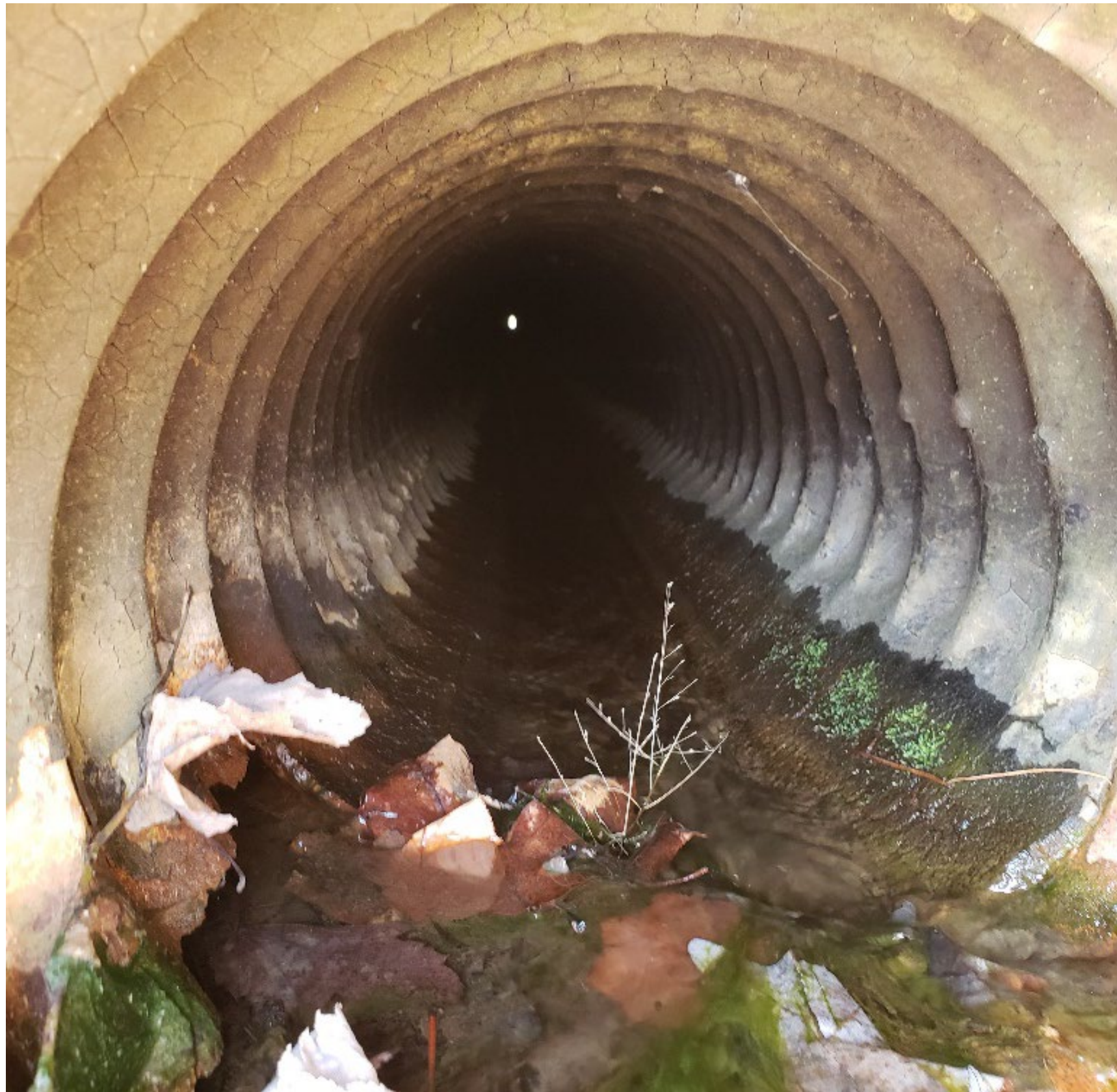
Deteriorated invert of a corrugated metal pipe culvert.
