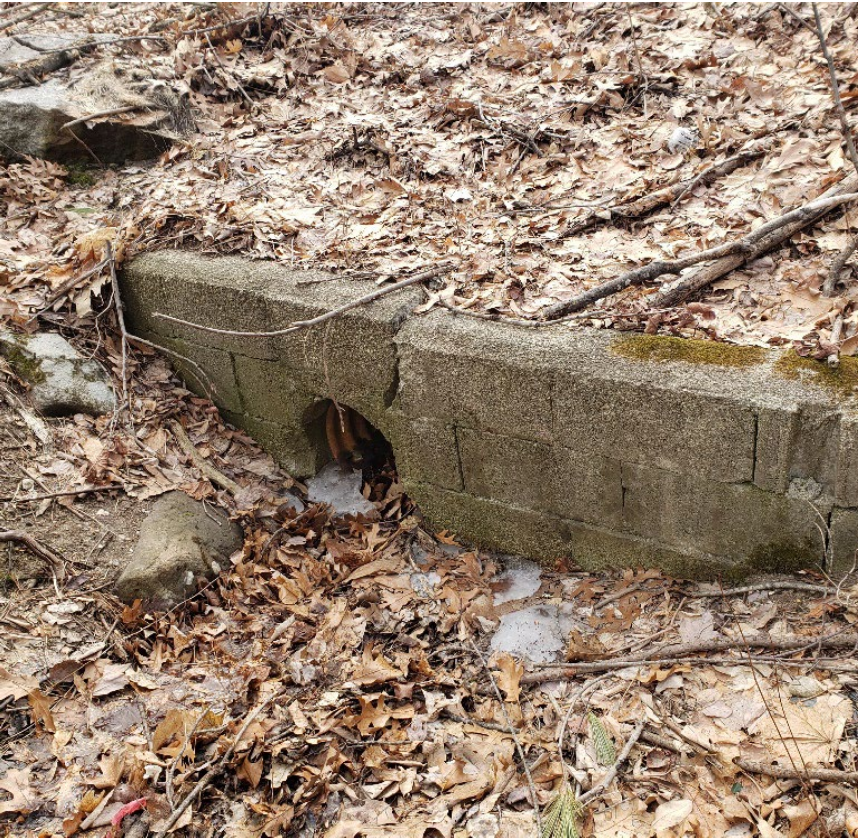
Existing headwall that is cracked at one of the stormwater outfall locations.
