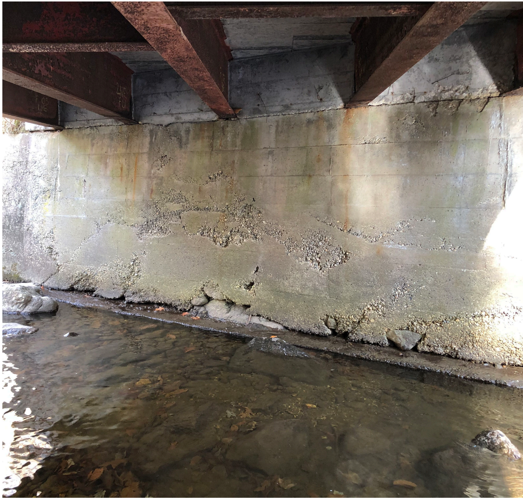
Scour Void Along the Base of the North Abutment
