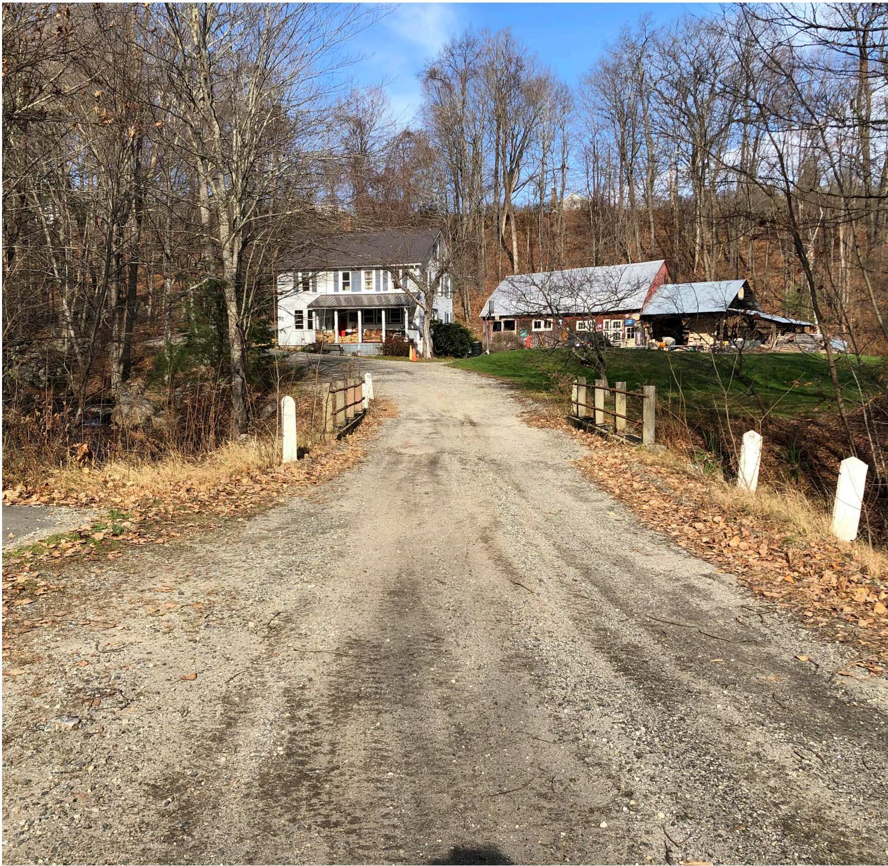
Looking North Across the Bridge - Missing and Outdated Guardrail
